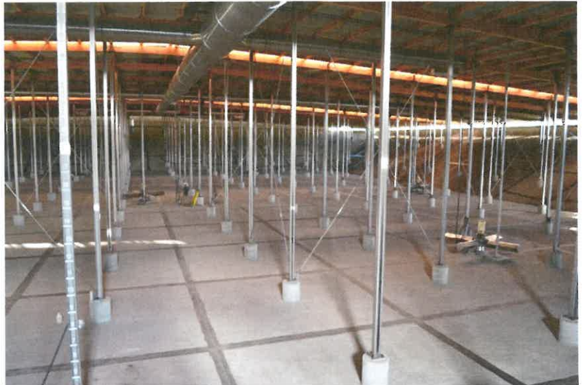
Empty tank – Empty More Ave. reservoir during installation of in-tank aeration system.
