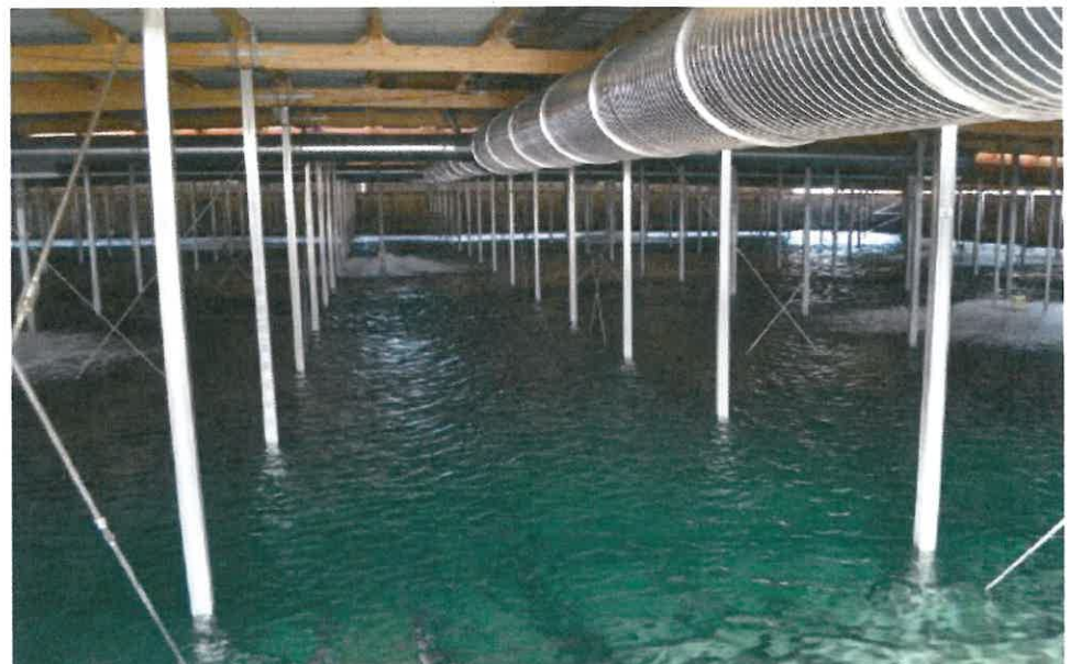
Filled More Ave. reservoir with in-tank aeration system in operation.
