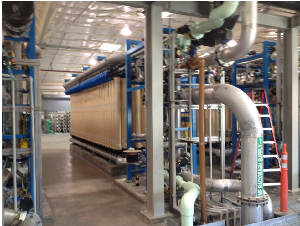
Figure 6-6: Pall MF System at the Existing SVAWPC
