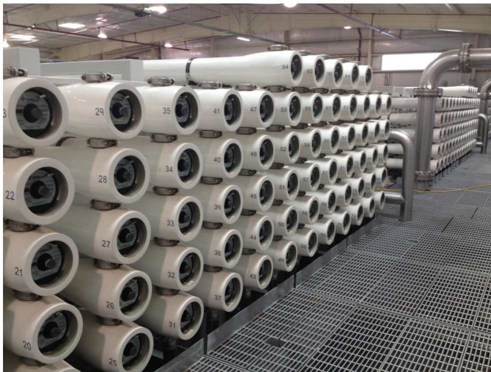
Figure 6-7: RO System at the Existing SVAWPC
