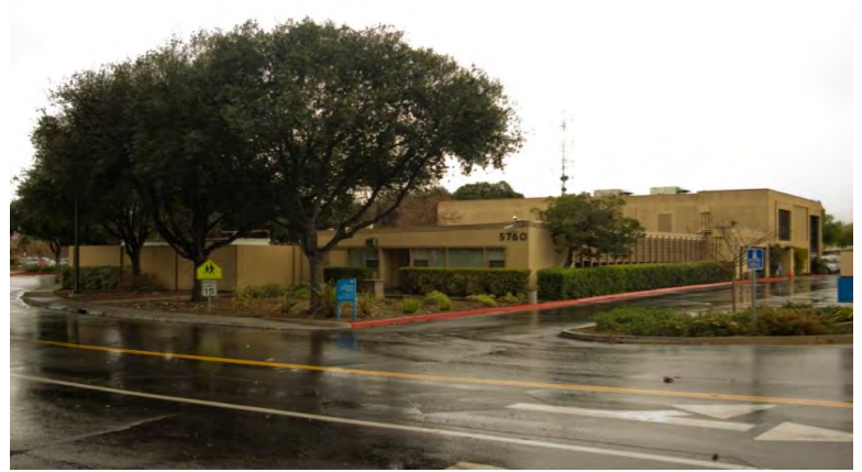
Existing Maintenance Building
