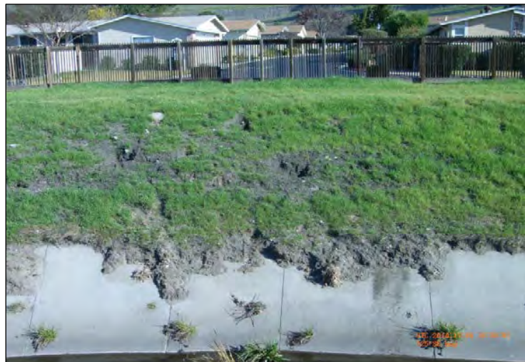
View of damage caused by burrowing animals along Canoas Creek in the Guadalupe Watershed
