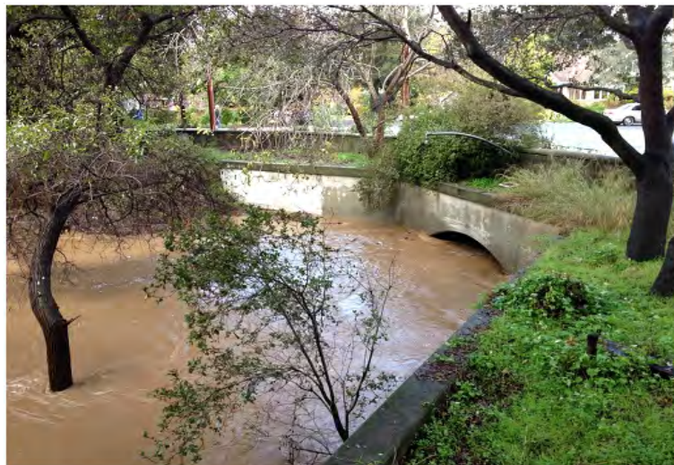
Upstream face of Pope/Chaucer Street with water surface approximately two feet below the soffit
