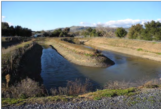
Main Avenue Ponds facing North
