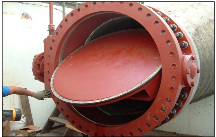
Valve installation in the Piedmont Line Valve Vault; Similar small capital projects will be carried out at treated water transmission facilities according to the asset management plan.
