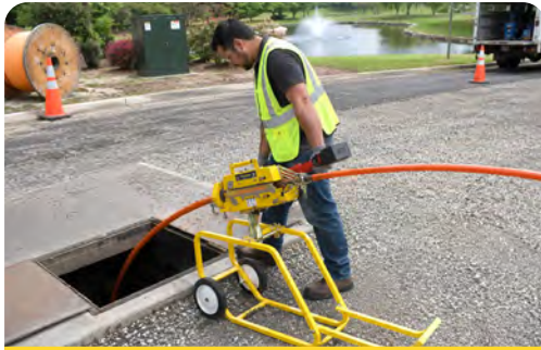
Utility Cable Installation
