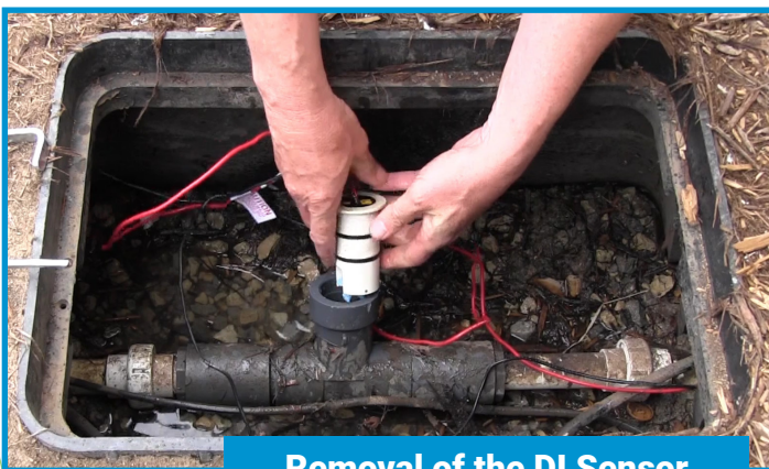
Removal of the DI Sensor
