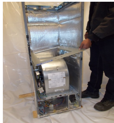
Figure 2: Coil Shelf Installation – Inserting Shelf
