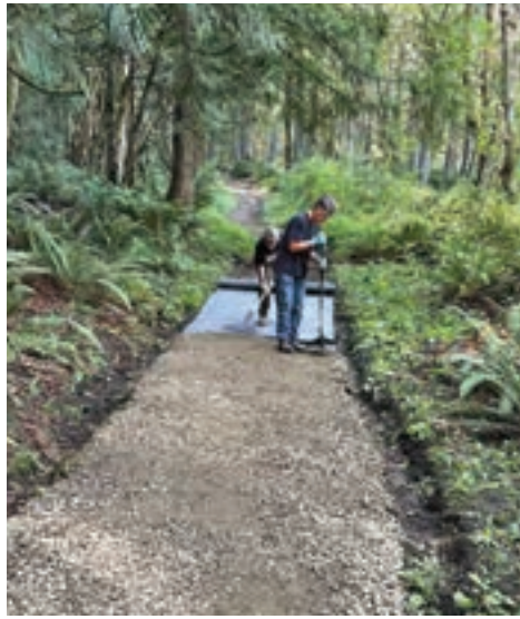
Board President Jane and her wife Cindy laying gravel on the multiuse trail at Chimacum Ridge Community Forest.
