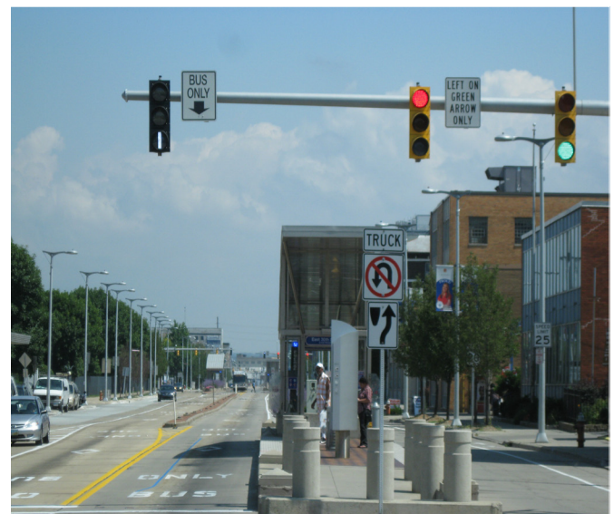
Dedicated, bus-only lanes with signal priority are typical ART system features.
