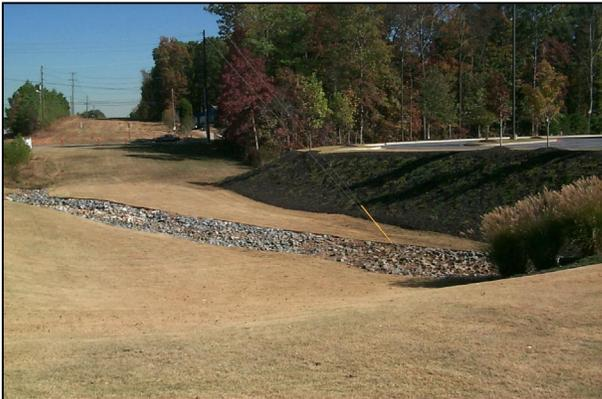
**Description:** A surface storage basin or facility designed to provide water quantity control through detention and/or extended detention of stormwater runoff.
