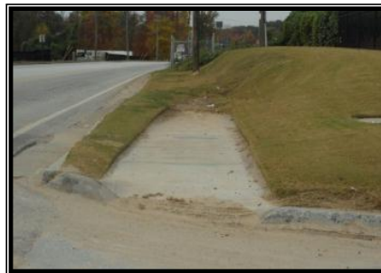
Lee Industrial Boulevard – Sidewalks damaged by truck turning
