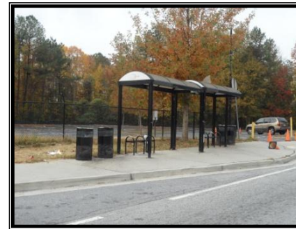
S. Service Road - Bus shelter with missing fiberglass siding.
