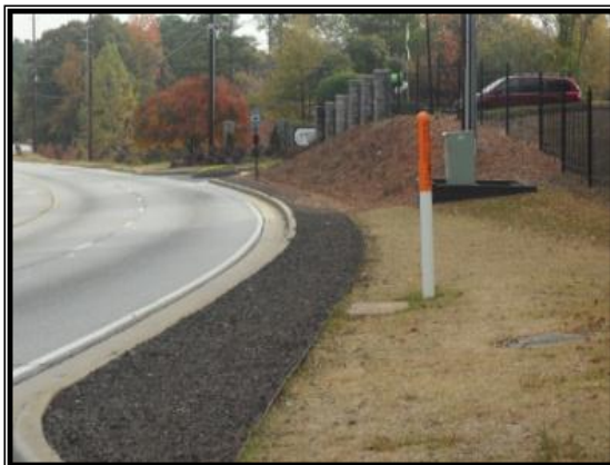
Six Flags Drive – Pedestrian path installed, but is flush with the curb, creating unsafe conditions.
