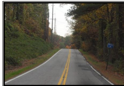
Factory Shoals – Narrow, patching, & worn edge of pavement.
