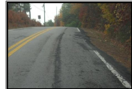
Factory Shoals – Narrow, patching, & worn edge of pavement.
