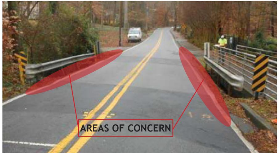
**During a recent inspection, it was determined that the outside sections of the Woodland Brook Drive Bridge over Gilmer Creek are in very poor condition. In order to maintain the structural integrity of the bridge until it can be replaced, traffic flow over the bridge is being reduced to one lane running through the center of the bridge.**
