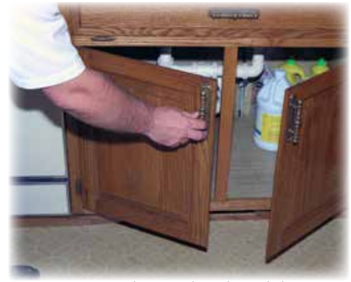
Opening cabinets under sinks can help prevent frozen pipes. Photo Source: https://tinyurl.com/w2bukpu
