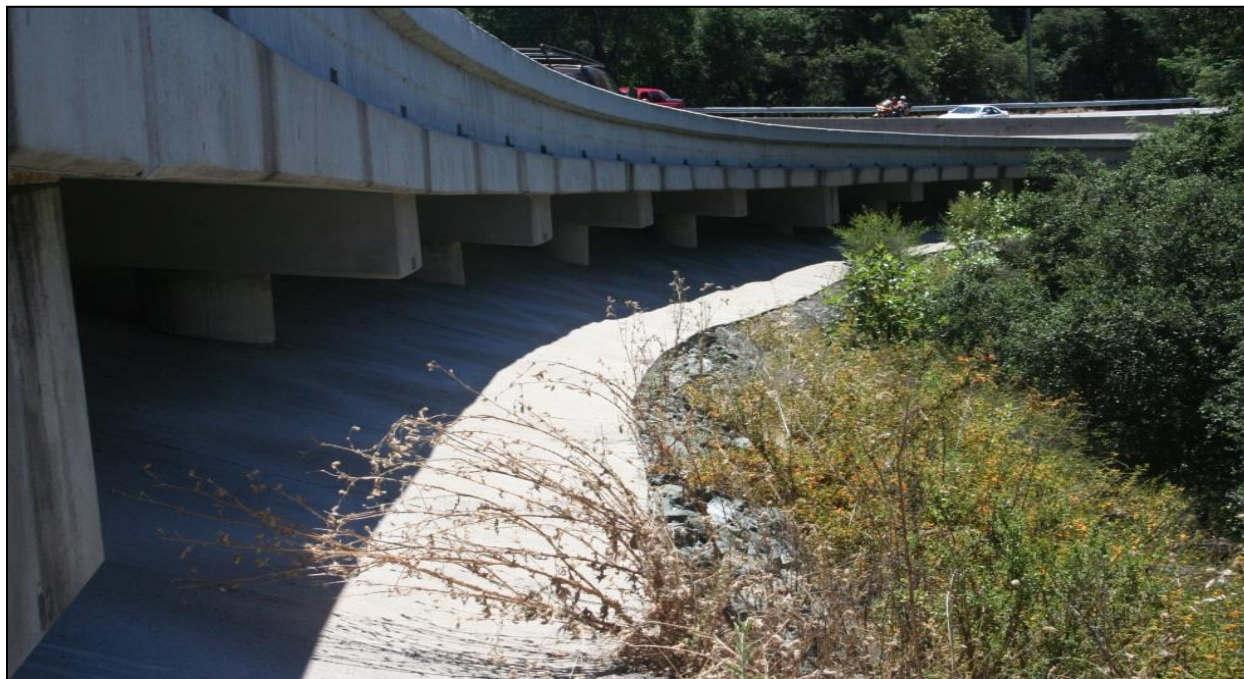
Figure 7. Cement wall viaduct at the Highway 17 Laurel Curve.
