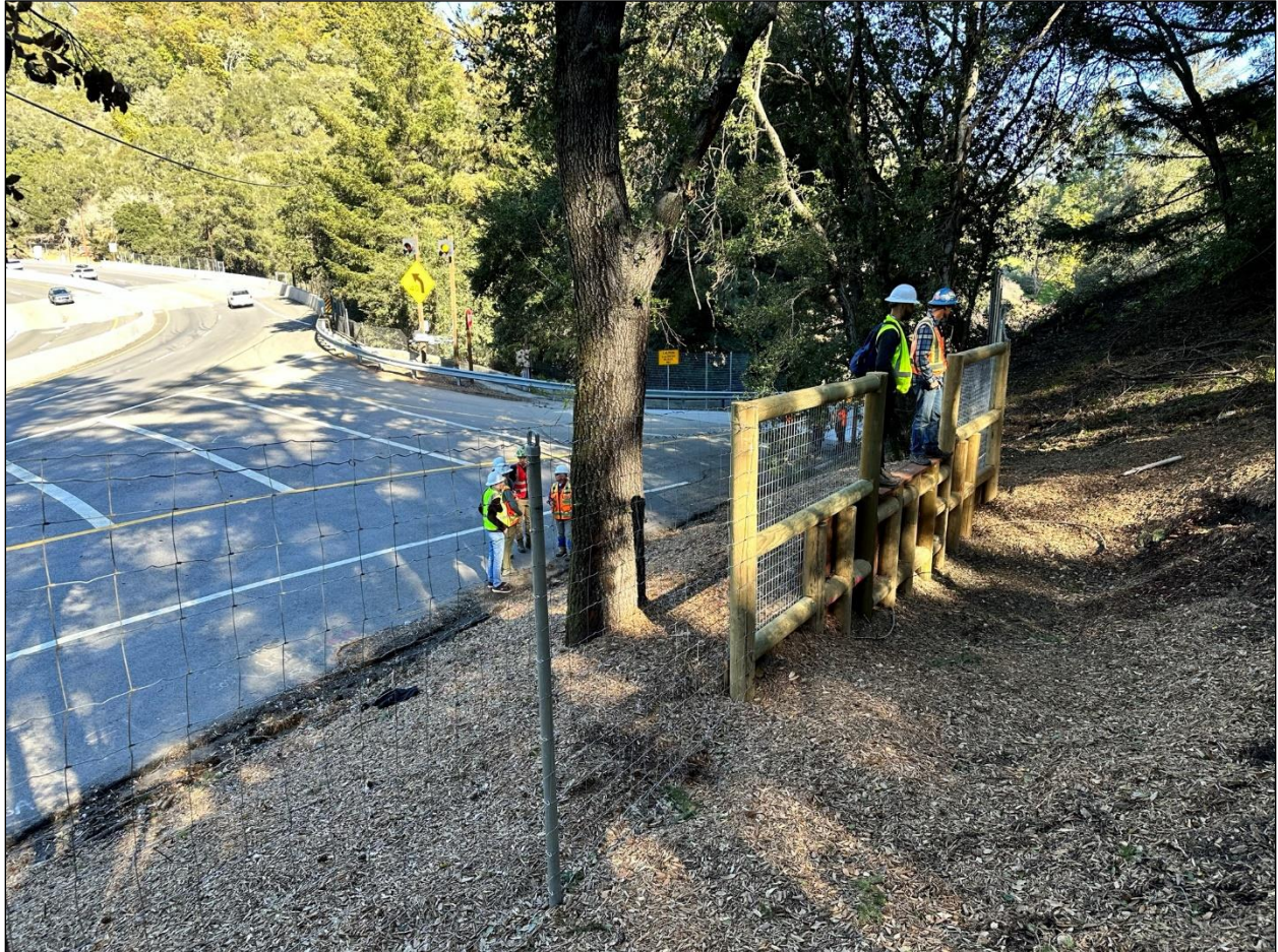
Figure 21. Highway 17 Laurel Curve exit jump-out with exclusionary fencing, south of the wildlife crossing.
