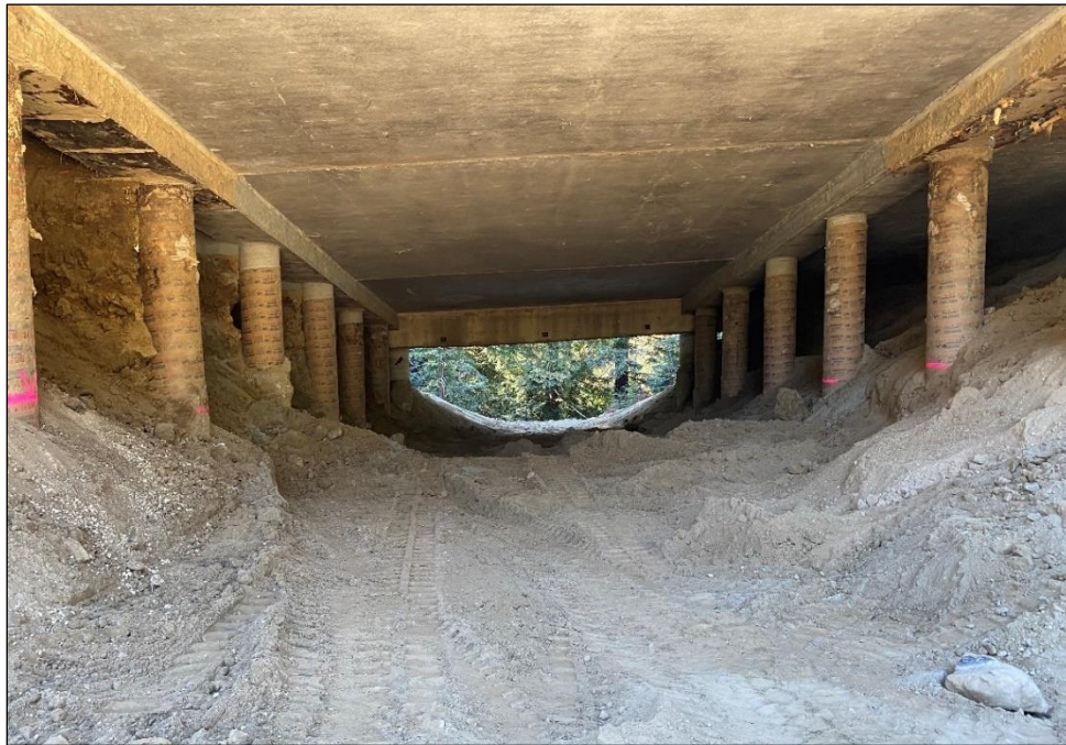
Figure 9. Post excavation of the Highway 17 Wildlife Crossing.
