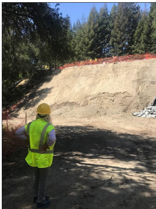
Figure 8. The fill dirt of the viaduct at the Highway 17 Laurel Curve.
