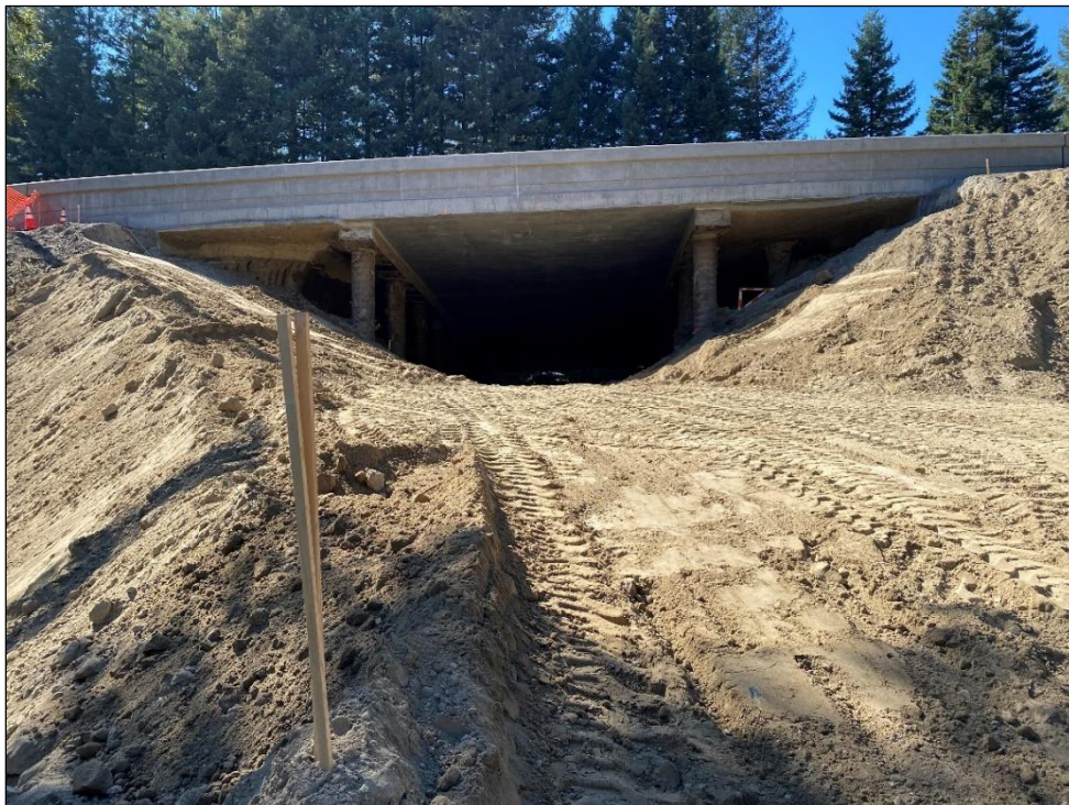
Figure 10. Post excavation of the Highway 17 Wildlife Crossing, east view.
