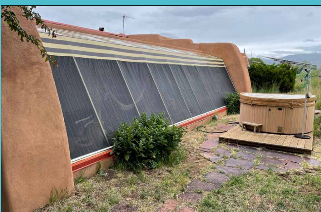
Here the inflated poly membrane has been replaced with the screen awning for summer. Two people can convert to the screen in an hour.
