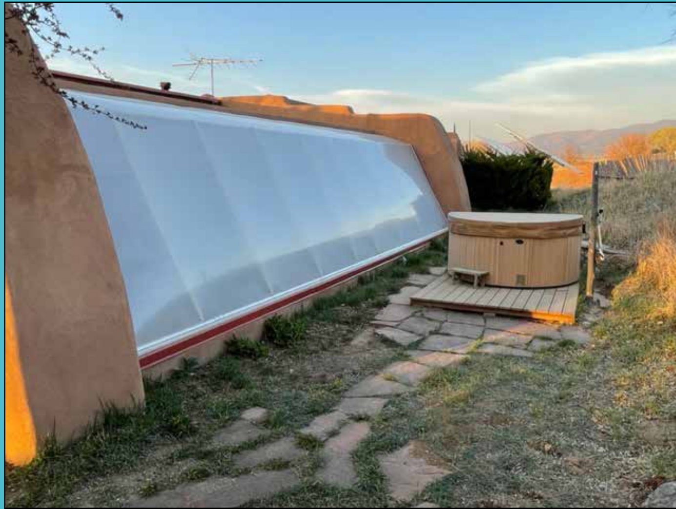
This 43 year old Solar Room® is the direct descendant of DOE-sponsored testing. It has an inflated polyethylene glazing membrane.
