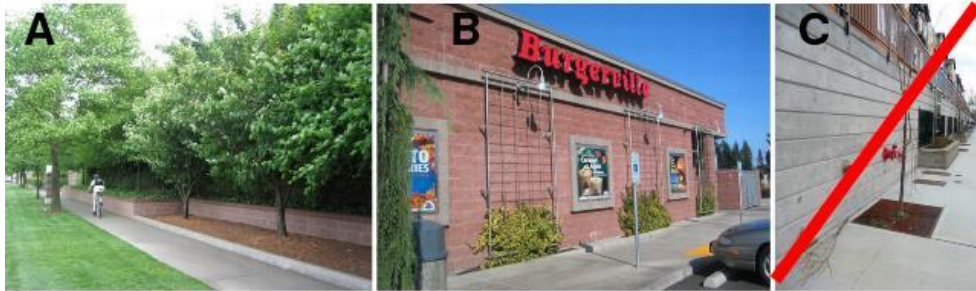
Figure 51. Good and bad blank wall treatment examples. Image A illustrates that heavy landscaping can be very effective in treating a large blank wall. Image B uses a combination of planted trellises and display ads integrated with the building's architecture along a facade facing a drive-through. Image C simply doesn't use enough treatments and the result is a stark and unwelcome streetscape.
