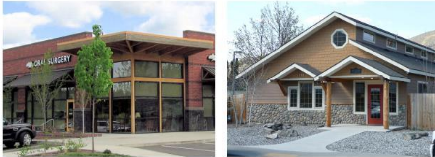
Figure 47. Acceptable facade detailing examples. The left image includes decorative window and roofline treatment on the corner plus decorative brick and stonework and metal awnings. The right image uses decorative stone and shinglework, decorative windows, and a decorative entry feature.
