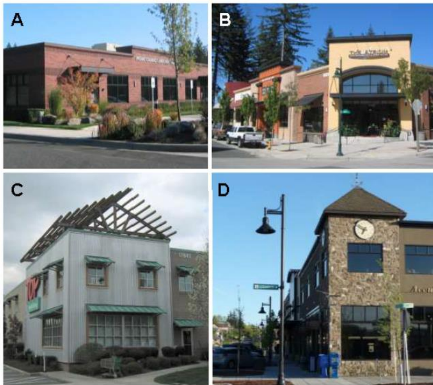
Figure 49. Acceptable mixes of building materials. Image A emphasizes brick; Image B mixes stucco, brick, and concrete block with metal weather protection elements; Image C mixes metal siding with heavy timbers; and Image D emphasizes stonework on the building’s corner.
