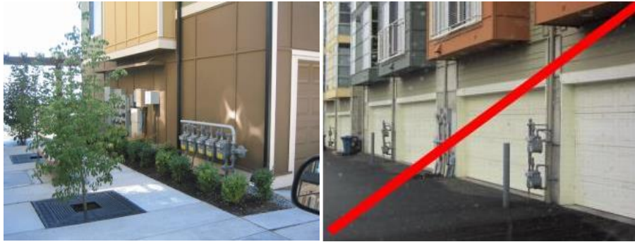
Figure 33. Good and bad utility meter configurations. The examples on the top are consolidated and somewhat screened by landscaping elements, whereas the bottom examples are exposed and degrade the character of these townhomes.
