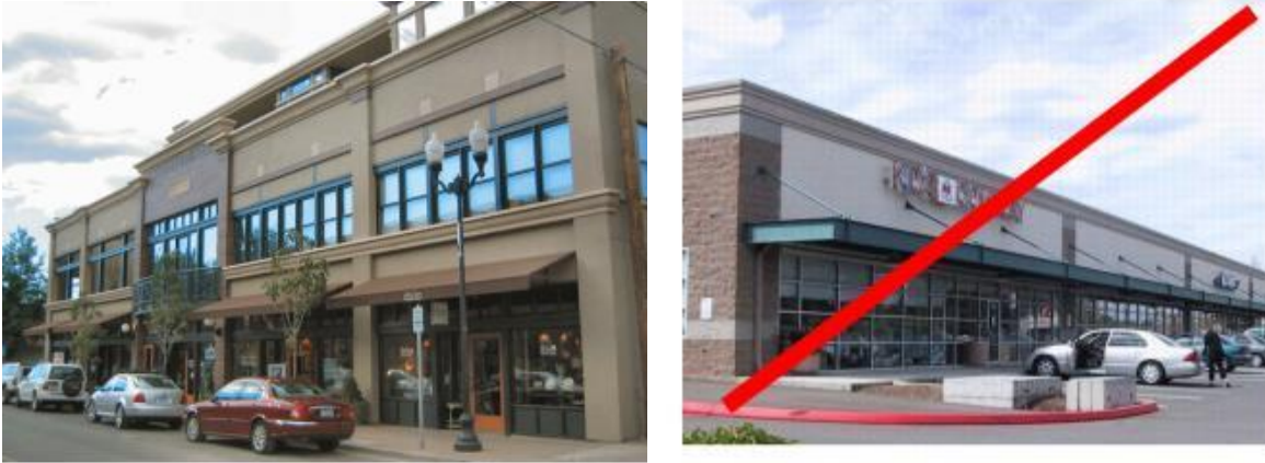
Figure 39. Facades that meet (top image) and don't meet (bottom image) the storefront articulation standards. The top image uses repeating window/storefront patterns, separate weather protection elements, and vertical piers to successfully articulate the facade. The bottom image uses continuous window and weather protection elements and thus wouldn't comply with the standards.
