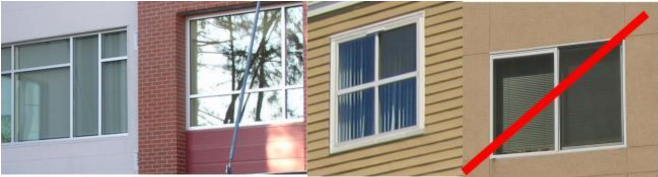
Figure 48. Acceptable and unacceptable (far right image) window design on upper floors. Note that the two windows on the left are recessed; the image right center shows a window with trim. The image on the right includes no trim or recess/projection.
