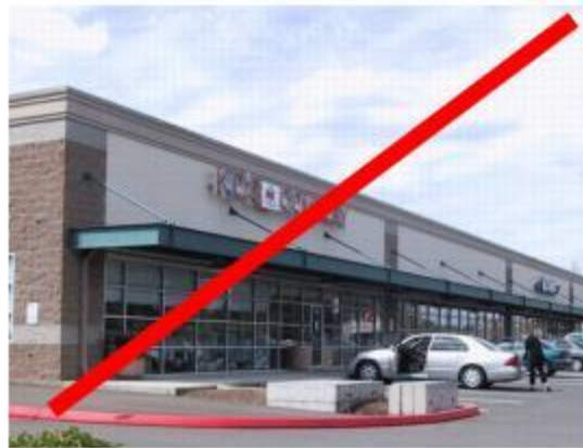
Figure 39. Facades that meet (top image) and don't meet (bottom image) the storefront articulation standards. The top image uses repeating window/storefront patterns, separate weather protection elements, and vertical piers to successfully articulate the facade. The bottom image uses continuous window and weather protection elements and thus wouldn't comply with the standards.
