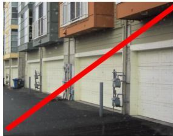
Figure 33. Good and bad utility meter configurations. The examples on the top are consolidated and somewhat screened by landscaping elements, whereas the bottom examples are exposed and degrade the character of these townhomes.
