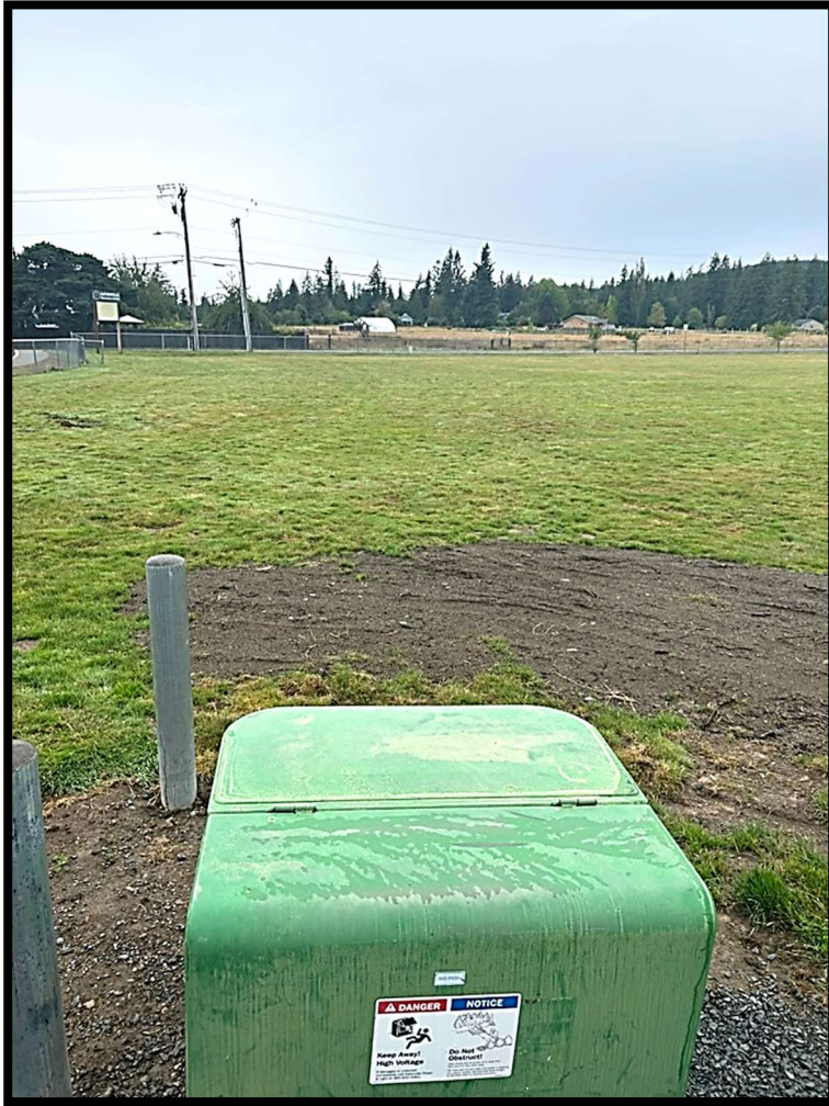
Left- Elementary School Portables Transformer in the foreground with repaired fault location behind it. The transformer is fed via a pole off Lynch seen in the background.
