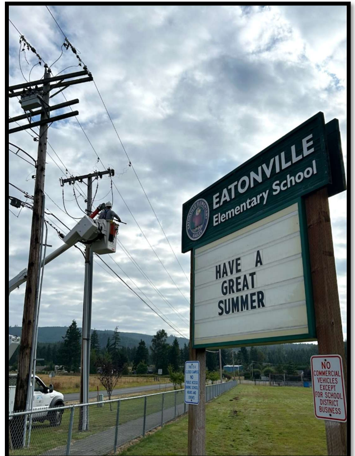
Right- Lineman restoring power after splicing out an underground fault
