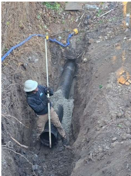
APP Fuel site stormwater pipe replacement
