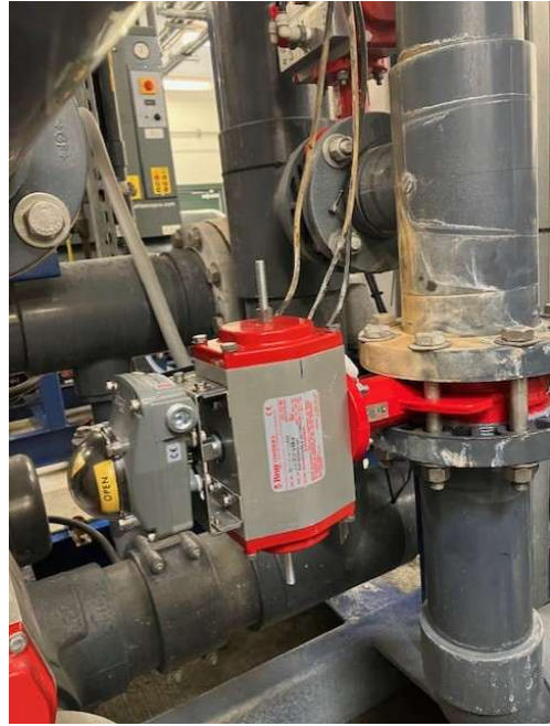
New valve and micro switch installed
