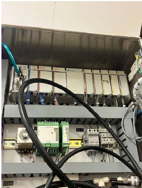
PLC output card replaced filter 2
