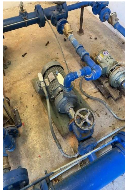
Finished installation of new booster
