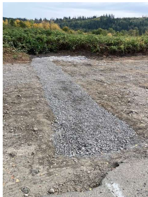
Completed Madison Ave Parking Area 'French Drain' drainage system
