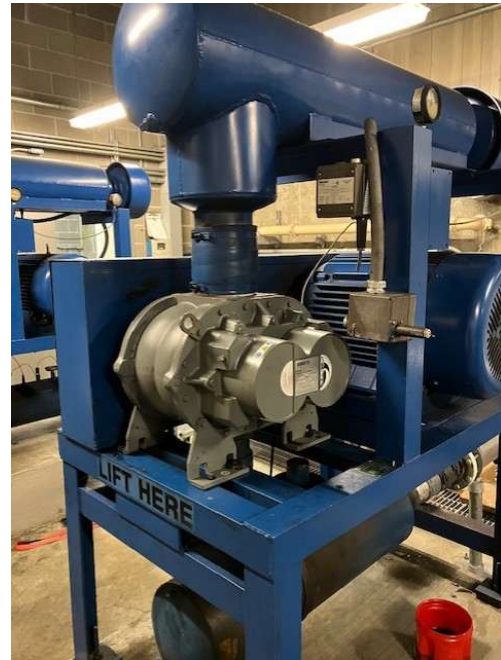
New blower installed at the Wastewater Treatment plant.
