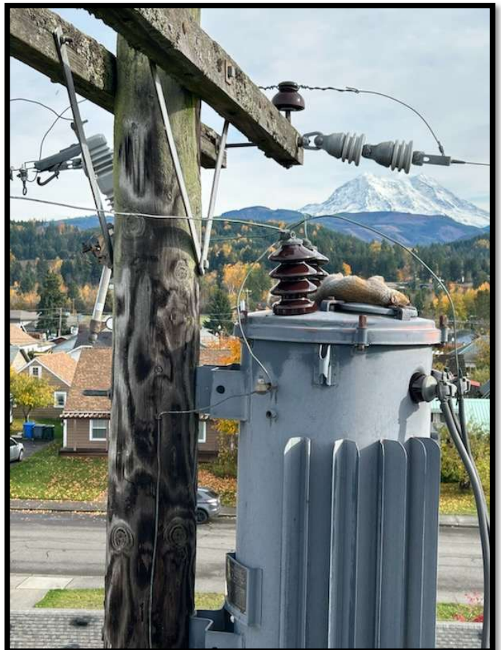
Squirrel on top of overhead transformer after contacting a live conductor and a grounded transformer in the 100 block of Orchard Ave N
