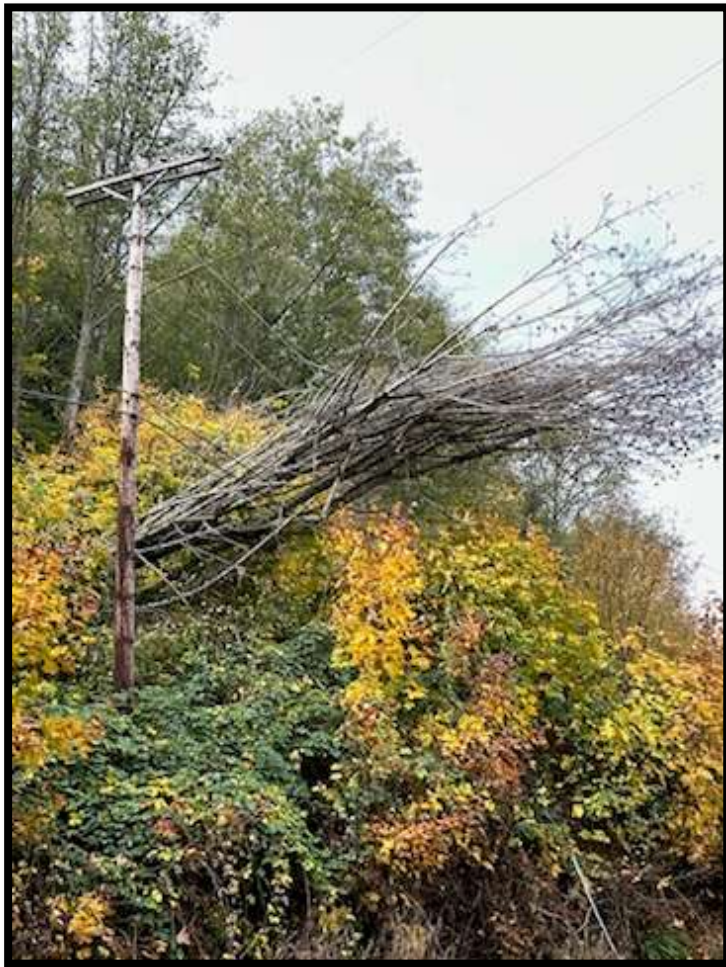
Group of trees on overhead feeder on 161
