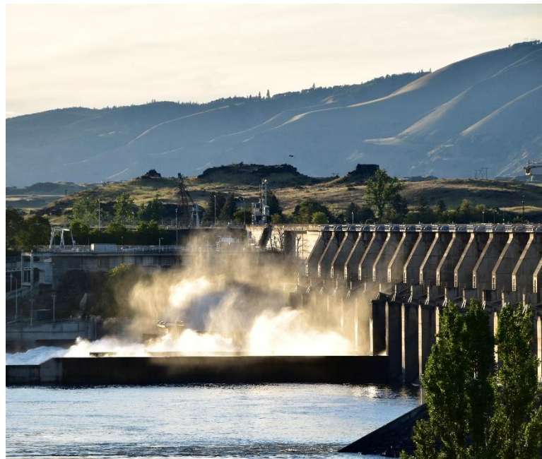
Spillway, The Dalles Dam
