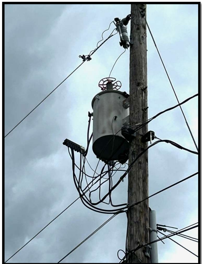
Overhead transformer pictured with “Zapshield” wildlife protection to save squirrels and nuisance outages
