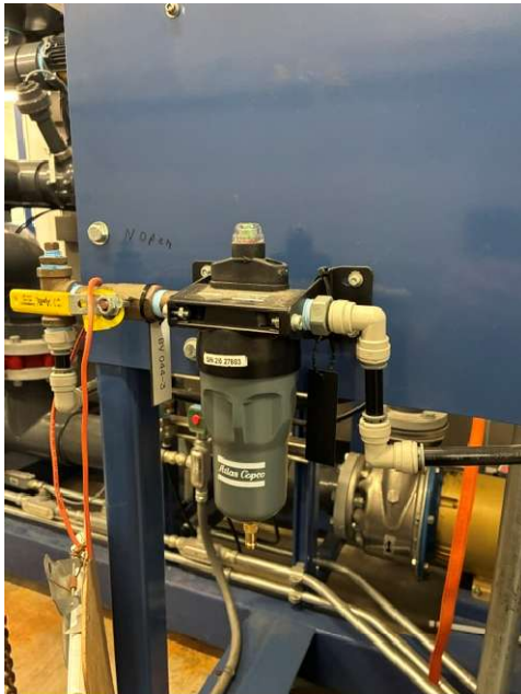
Rebuilt air separator filter 3 water plant
