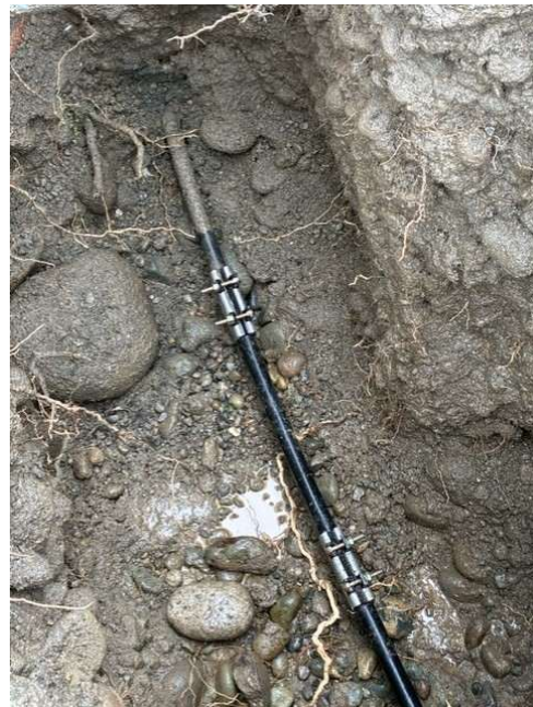
Water Repair Antonie Ave N
