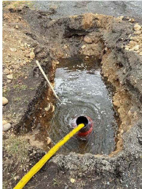
Water drainage test Ridge Rd
