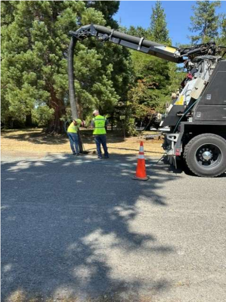
Potholing to locate water main Ridge Rd
