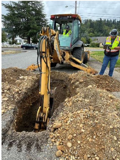
Soil test Penn Ave N
