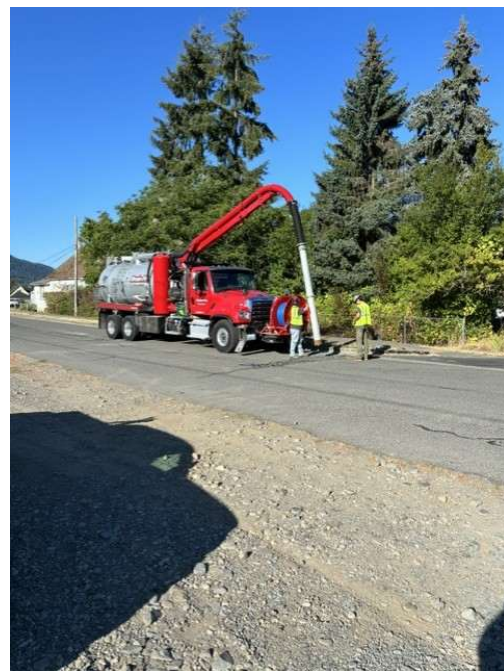
Stormwater cleaning on Madison Ave
