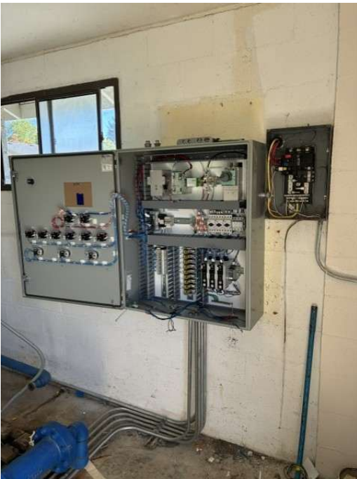
Telemetry Panel Install Center St Pumphouse
