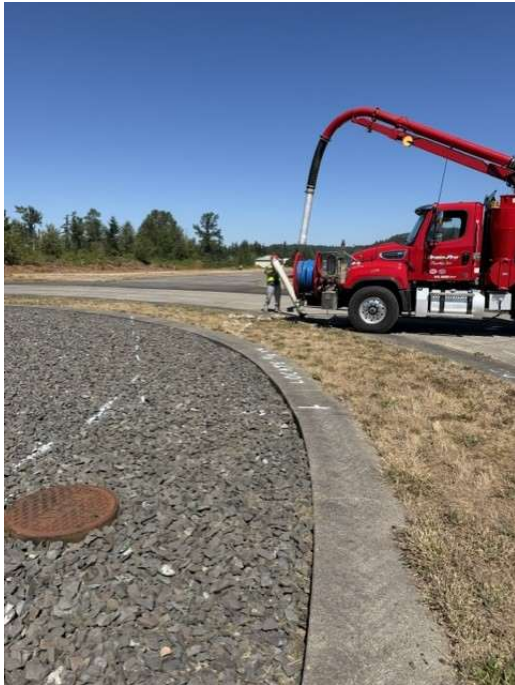
Potholing to locate stormwater pipe near the airport
