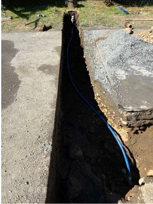
Water Service Line Replacement Fir Ave N
