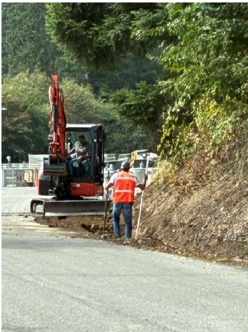
Stormwater ditch in yard
