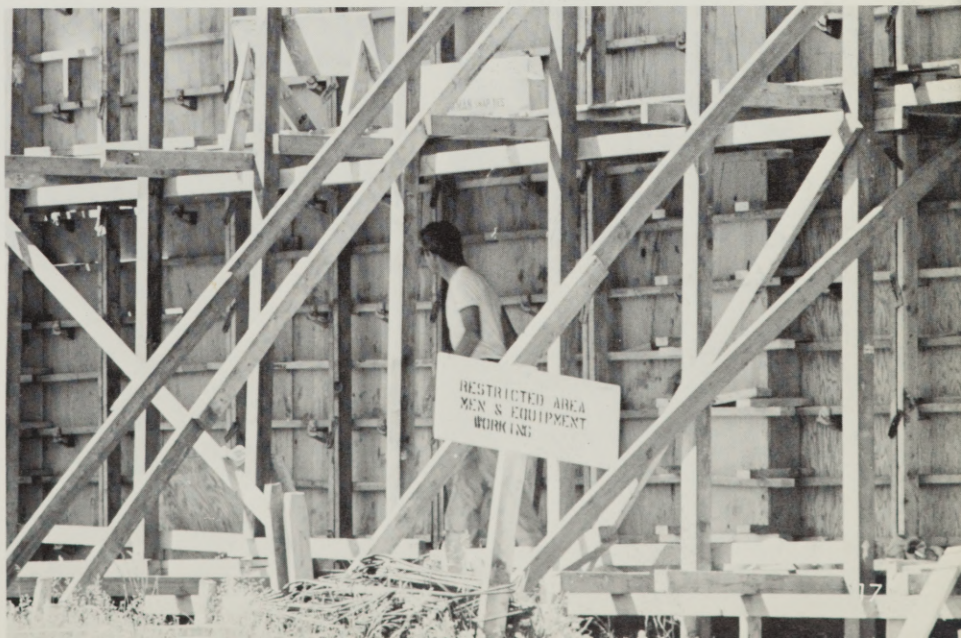
Below- The new swimming pool is starting to take shape.
