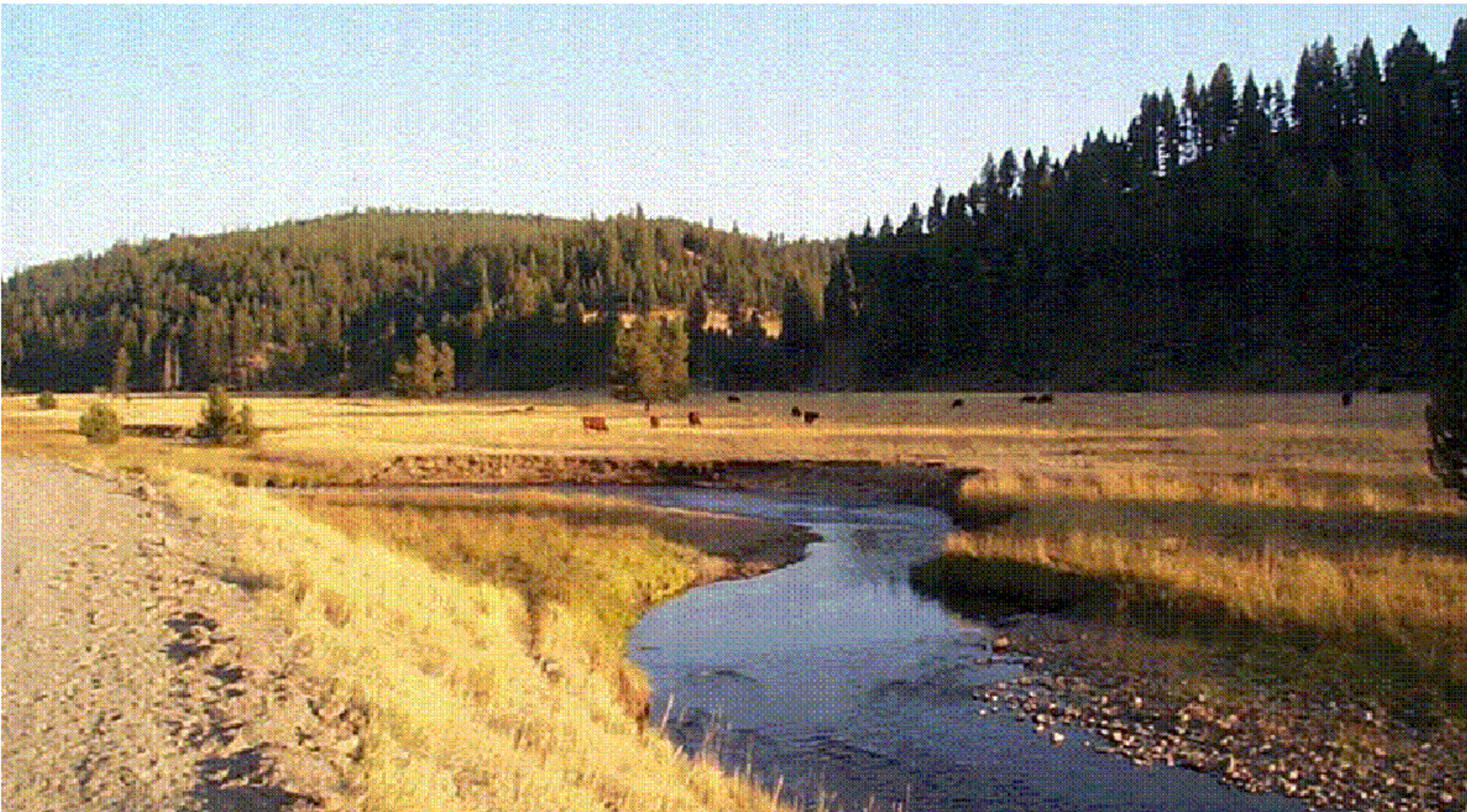
Poor shade results from near stream vegetation removal and is compounded by channel morphology response to near stream vegetation removal (Vey Meadow, Grande Ronde River, Oregon)
