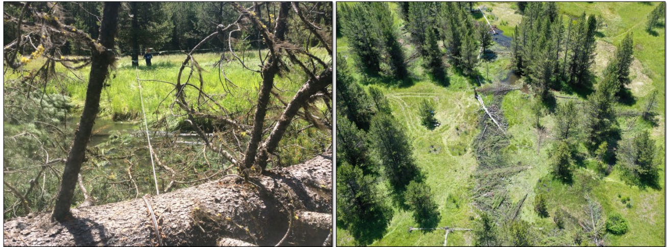
Figure 13. Utilizing a griphoist to move large wood from the adjacent floodplain into the stream channel (left photo) and example of high densities of large wood left unanchored in the channel and placed on the floodplain to add roughness (right photo). Photo examples are from restoration on a tributary to the upper Grande Ronde River in Oregon.
