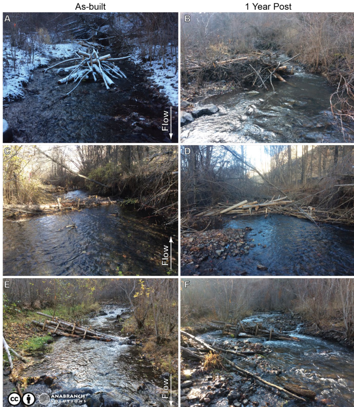
Figure 22. Example of PALS evolution over the course of one year promoting processes of wood accumulation. A and B show a mid-channel PALS becoming a bank-attached PALS, C and D show a bank-attached PALS becoming a debris jam, and E and F show a bank-attached PALS becoming a mid-channel PALS. The geomorphic changes imposed by the presence of the PALS in each example shows clear alterations to the channel bed and hydraulics. From Chapter 4 of Wheaton et al. (2019: http://lowtechpbr.restoration.usu.edu ).
