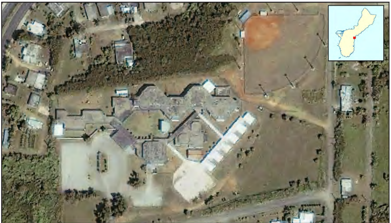
M.U. Lujan Elementary School Guam
