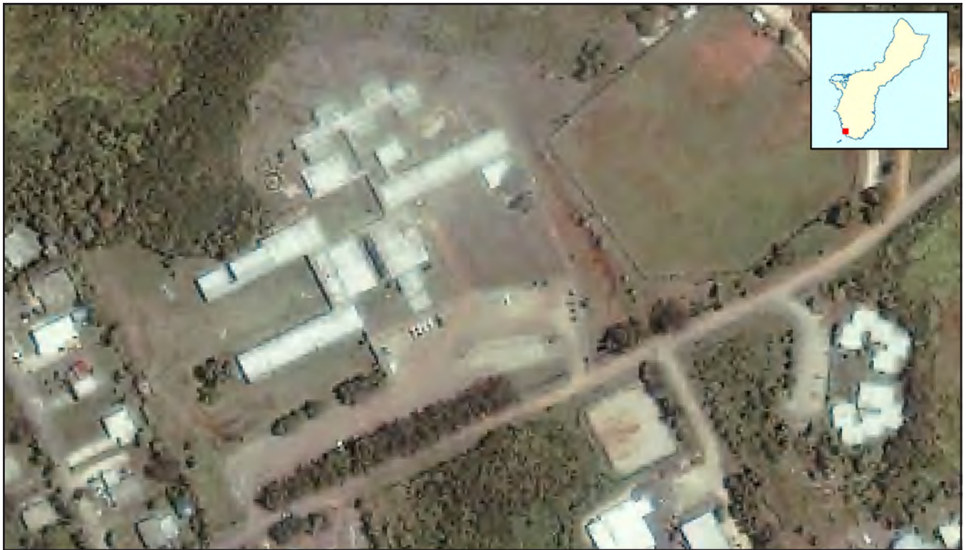
Merizo Martyrs Memorial Elementary School Guam
