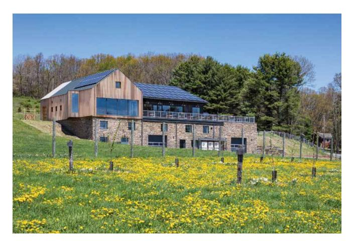
Overlooking the orchard, the cidery combines a ground-floor production facility with a top -floor tasting room and event space. The wood inside and outside the cidery is larch reclaimed from the underwater pilings of the old Tappan Zee Bridge.
