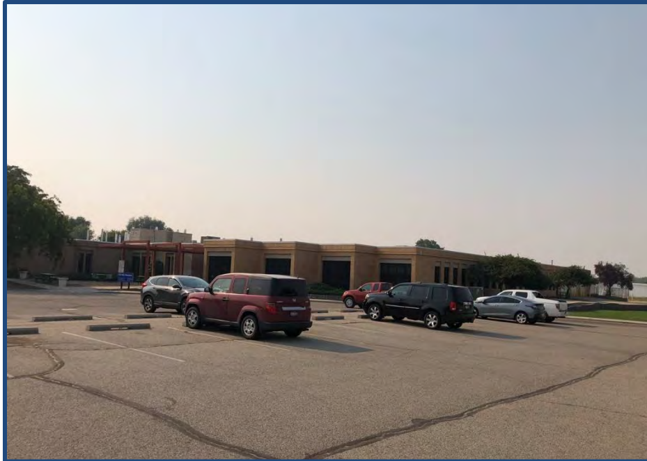
Operations Annex Building
