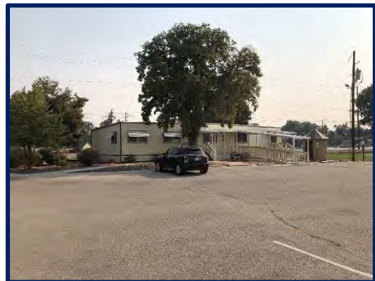
Modular Building - ETS
