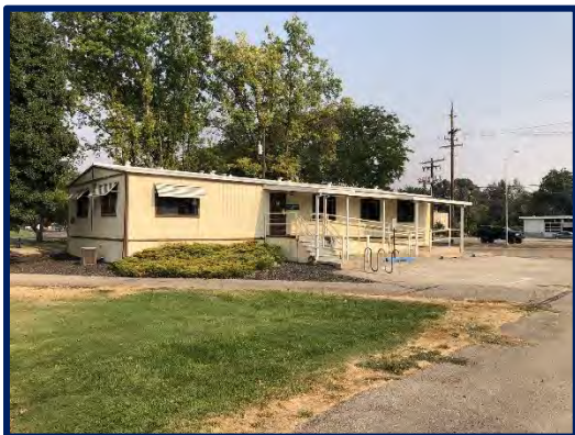
Modular Building - Training
