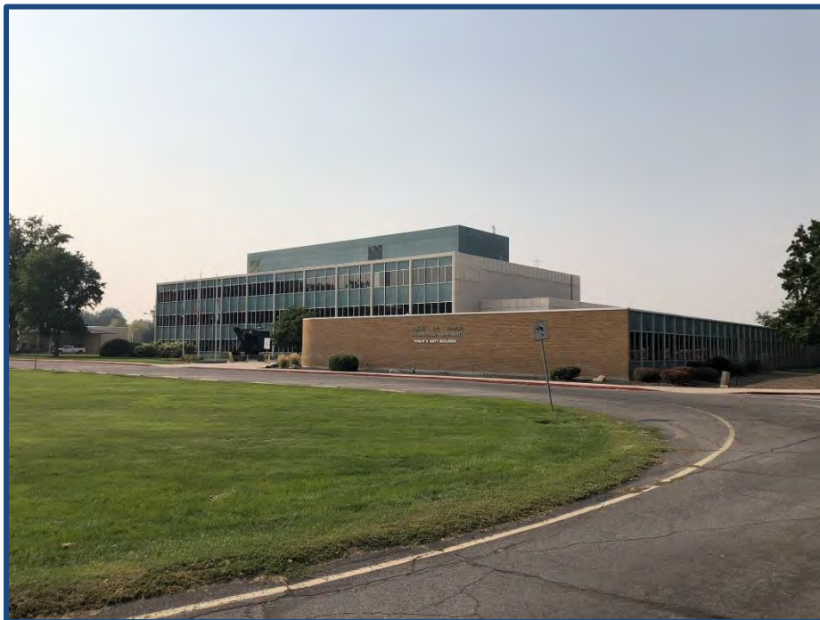
ITD Headquarters Office Building
