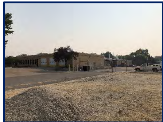
Operations Annex Building rear
