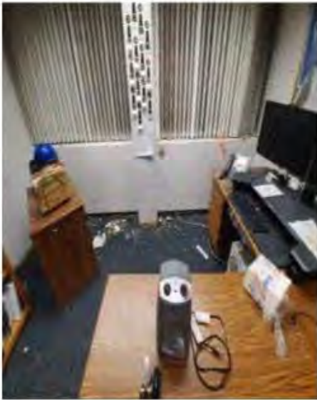
9) Impacted office area with visible debris.
