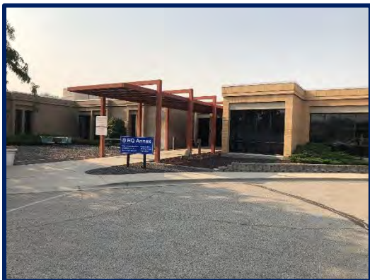
Operations Annex Building front
