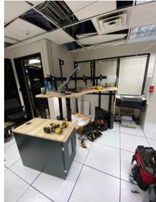
Xybix console installation in progress at Clallam County Jail. We consider ergonomics and human factors to be an important element of control center design, for officer comfort and mitigation of repetitive stress injuries.
