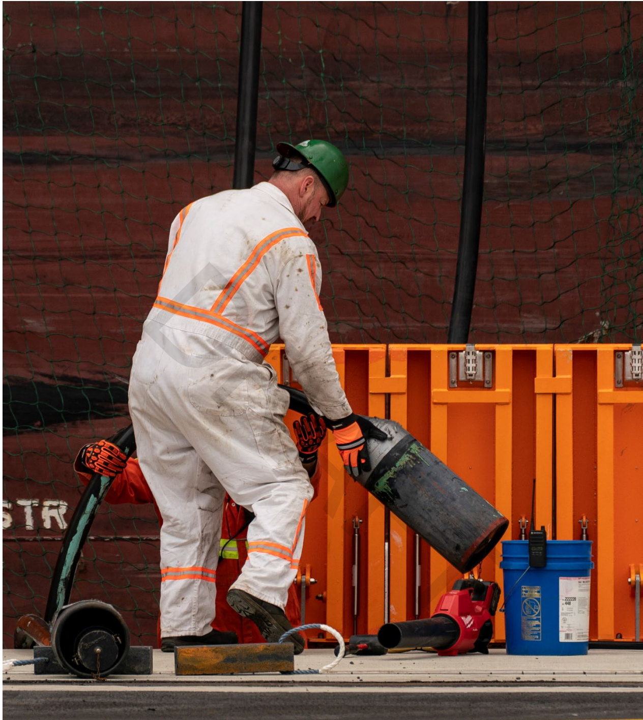
Longshore worker connecting an MSC vessel to shorepower at Terminal 5 in the North Harbor.
