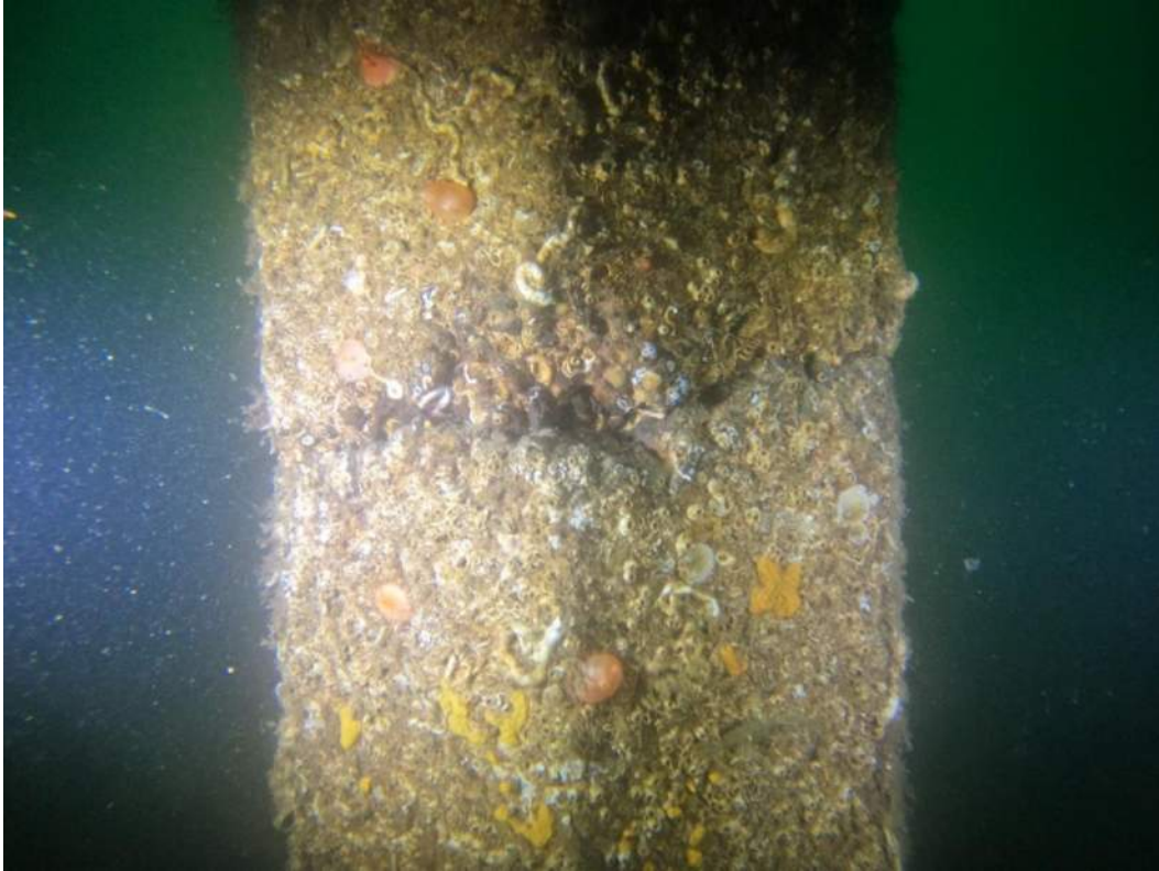
Photo 16: Pile 26:G, Major Tension Crack with Spalling
