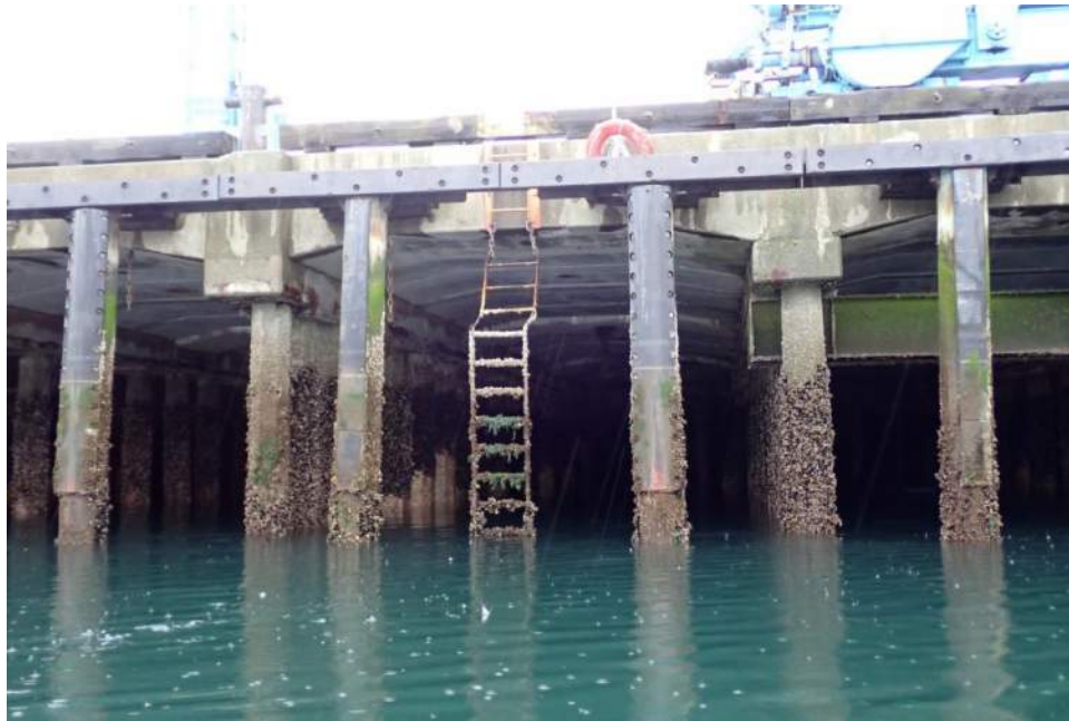
Photo 2: Typical Fender System
