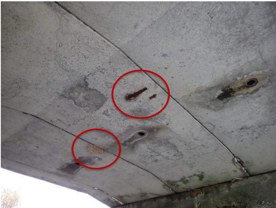
Photo 13: Typical Minor Deck Panel Spalling and Corrosion Staining
