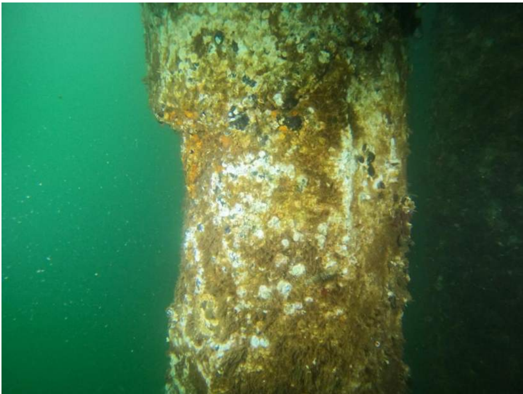
Photo 17: Pile 26:A, Severe Spalling with Section Loss
