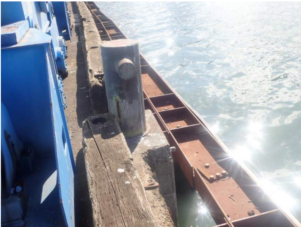
Photo 9: Typical Mooring Bollard
