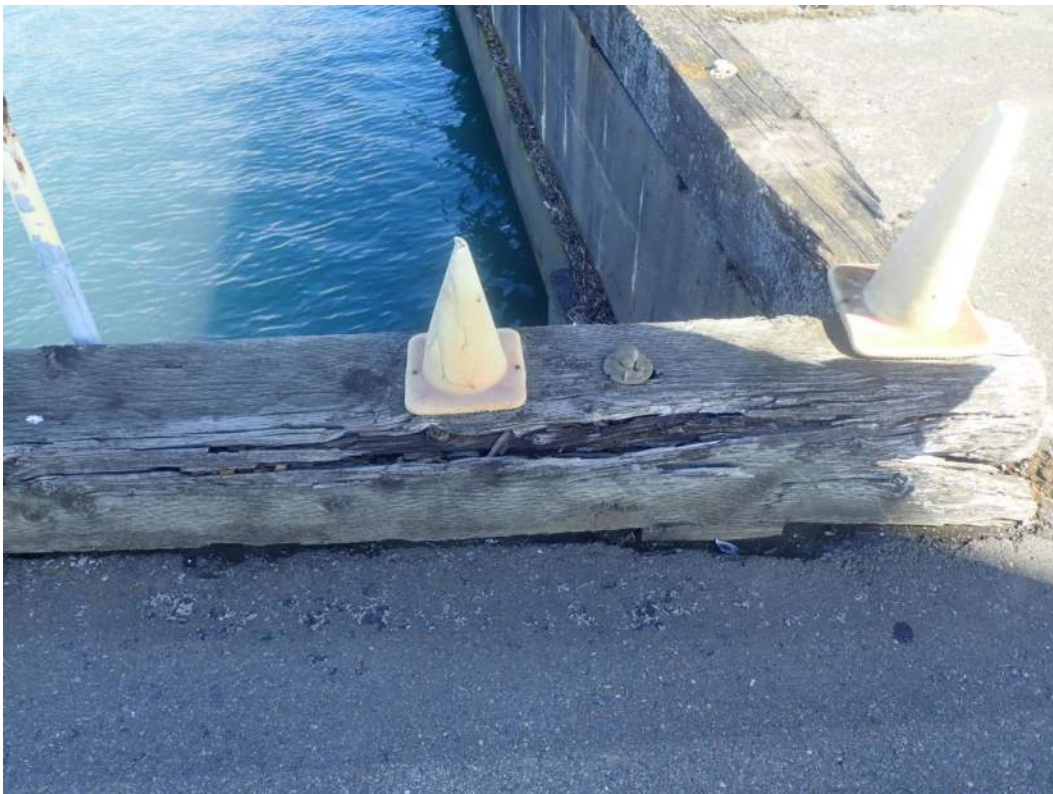
Photo 7: Typical Moderate Bullrail Decay
