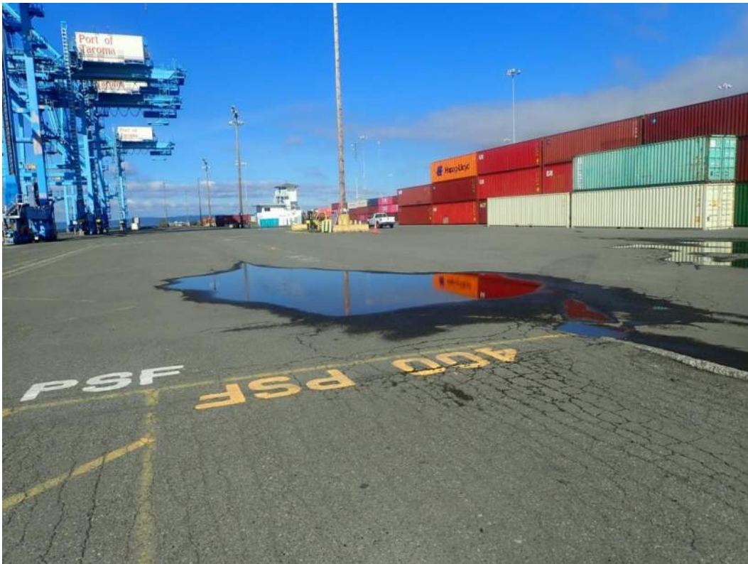
Photo 5: Deck Ponding from Bent 1 to 3
