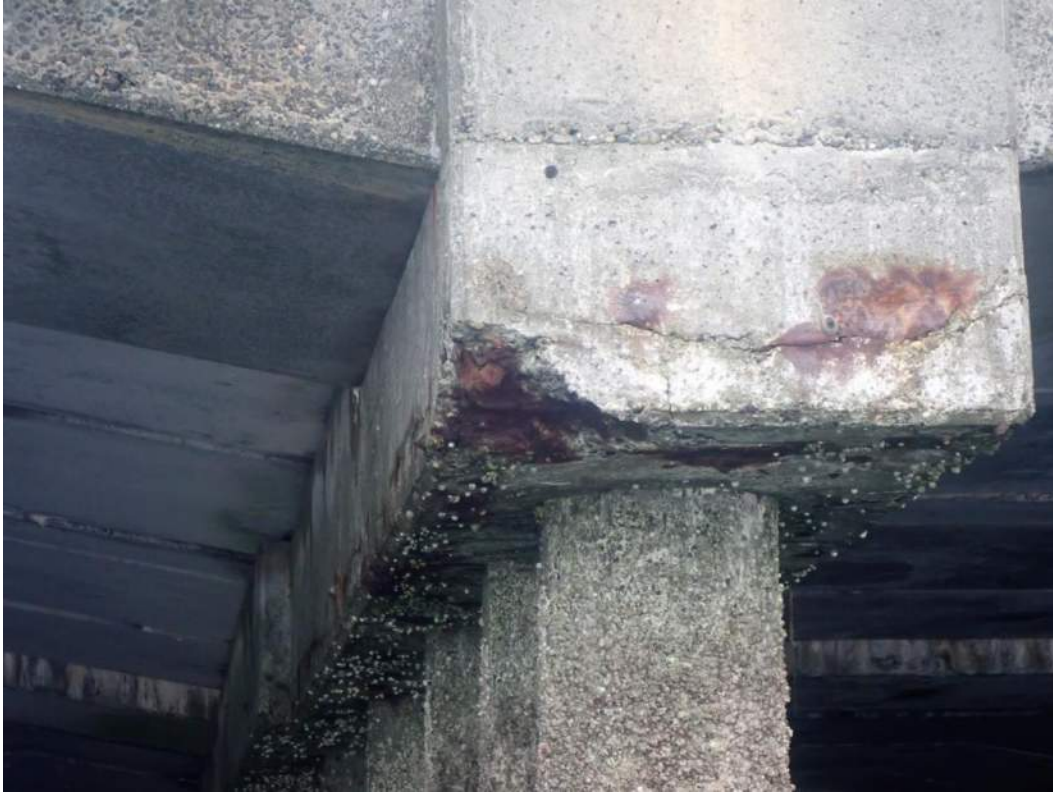
Photo 14: Typical Pile Cap Spalling with Exposed Rebar
