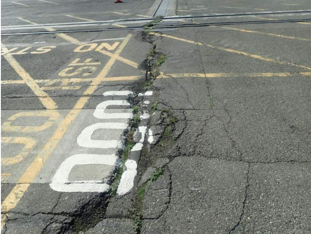
Photo 6: Berth C to Berth D Transition Asphalt Overlay with Cracks and Potholes
