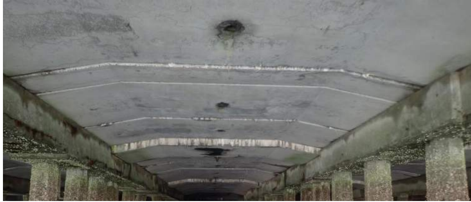
Photo 1: Typical Below-Deck Framing
