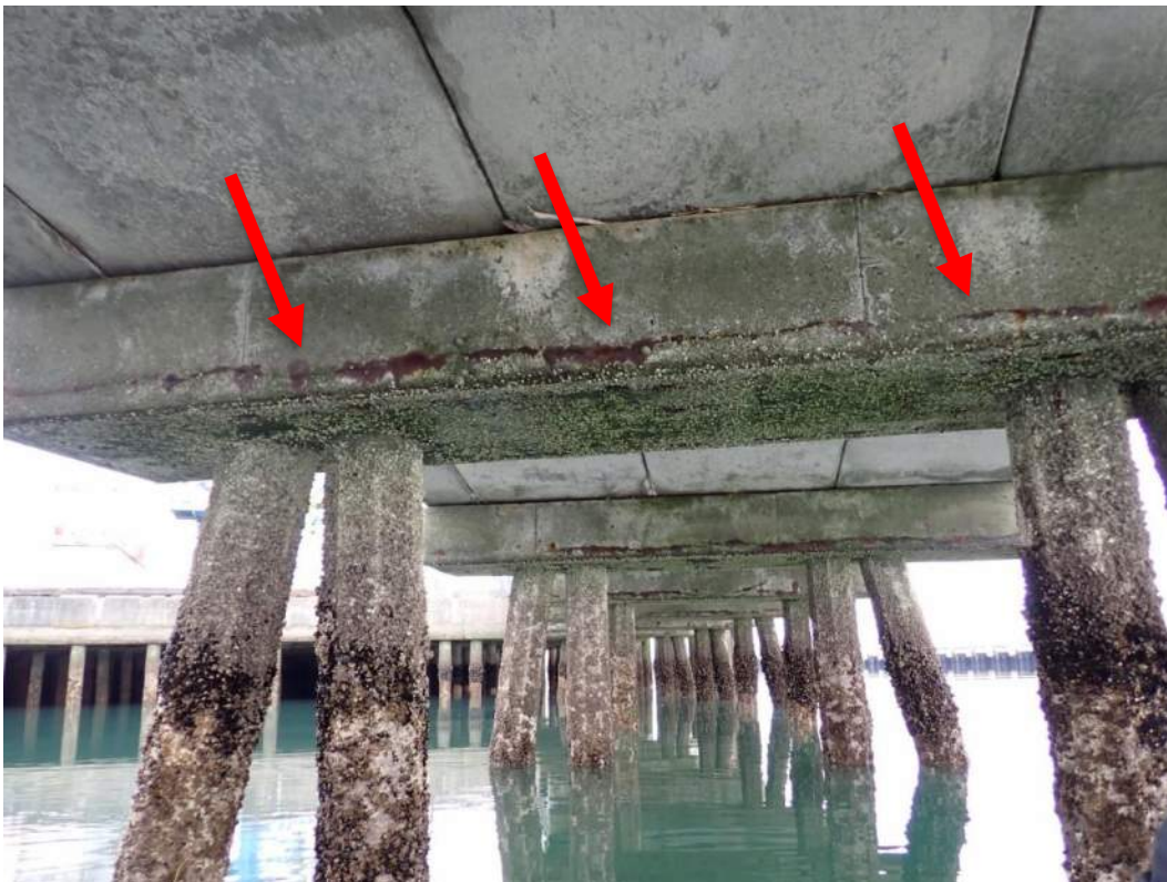
Photo 15: Typical Pile Cap with Corrosion Cracks
