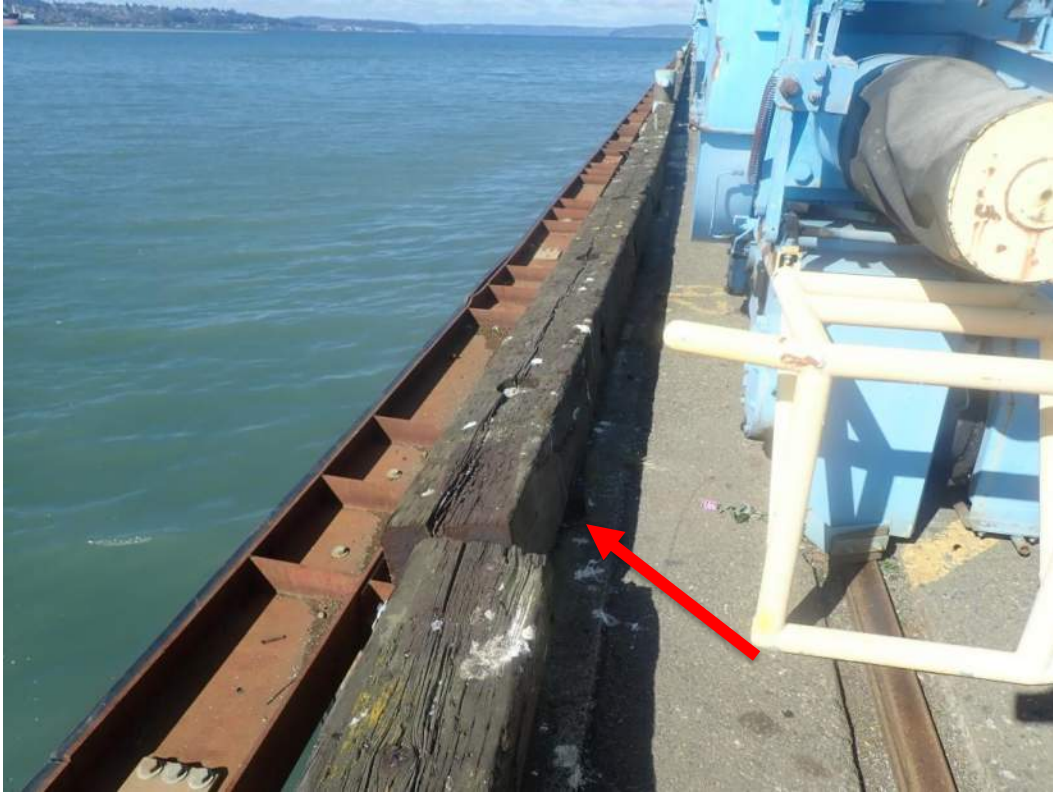
Photo 8: Bullrail Missing Hardware, Not Secure
