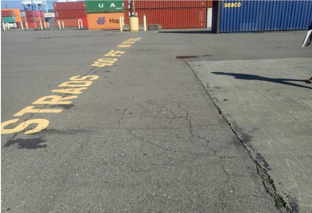
Photo 4: Asphalt Overlay with Map Cracking
