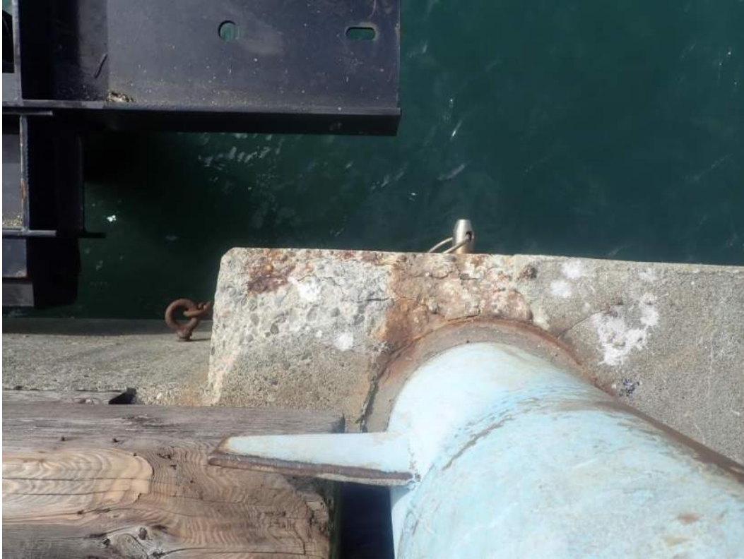
Photo 10: Typical Minor Spalling with Cracks at Mooring Hardware Foundation
