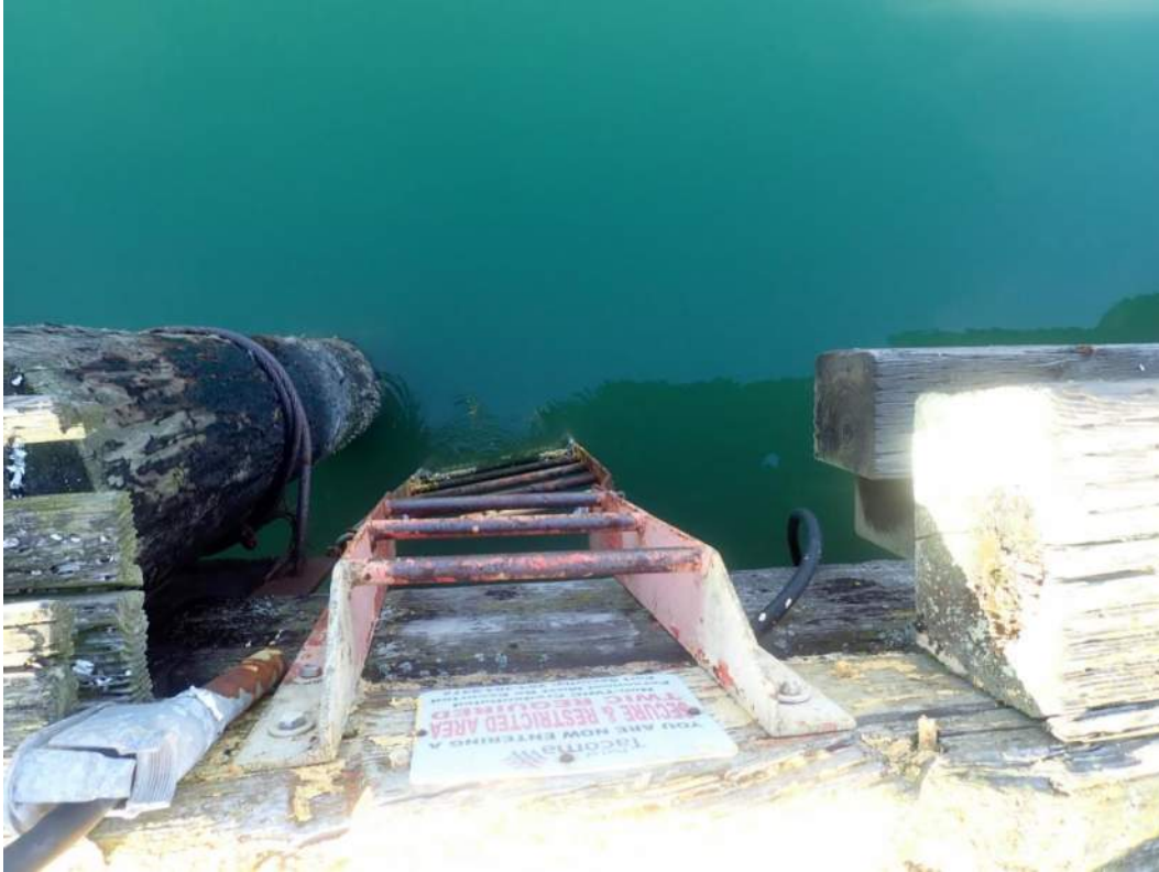
Photo 12: Typical Ladder with Impact Damage and Surface Corrosion
