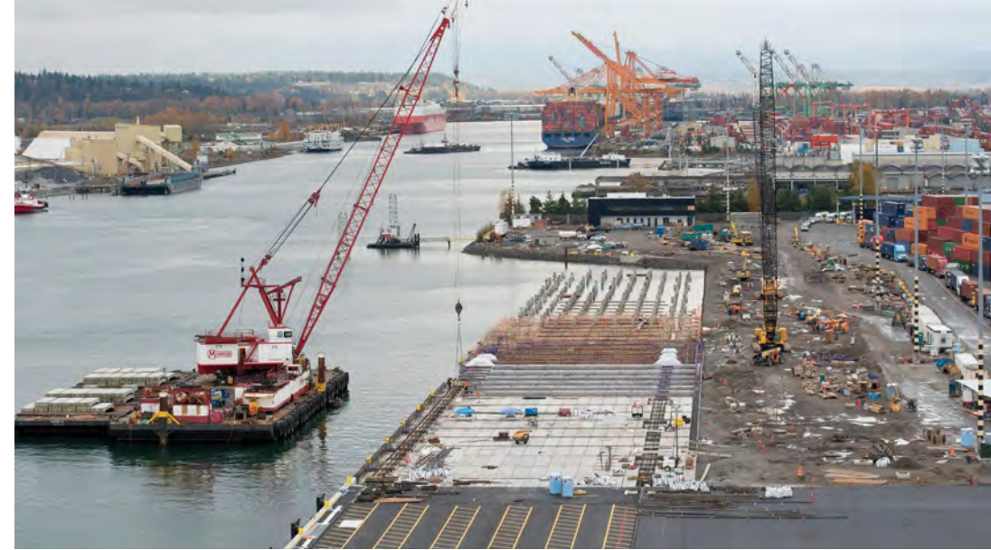
Crews drove 1,245 piles into the Blair Waterway at Pier 4 as part of the $250 million terminal improvement project.
