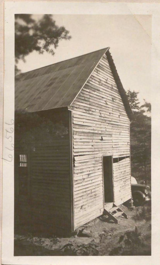
Scott's Creek Church - 1940
