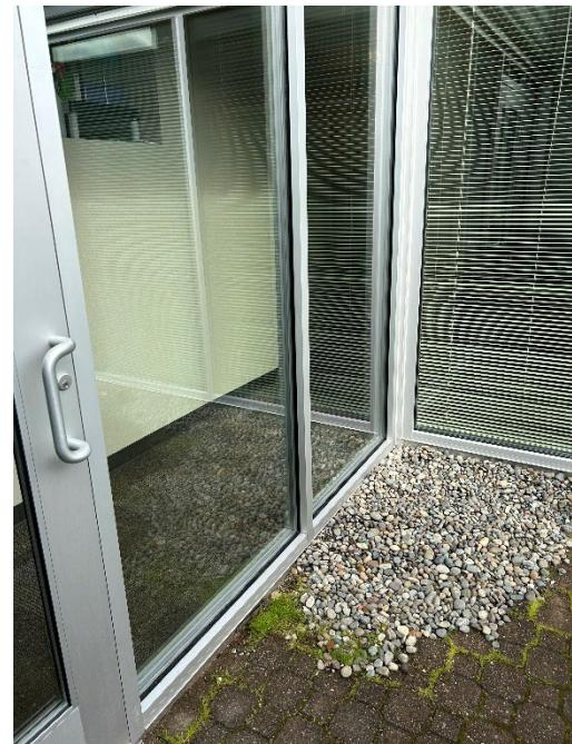
Figure 2 - After construction, new sealed aluminum storefront window system
