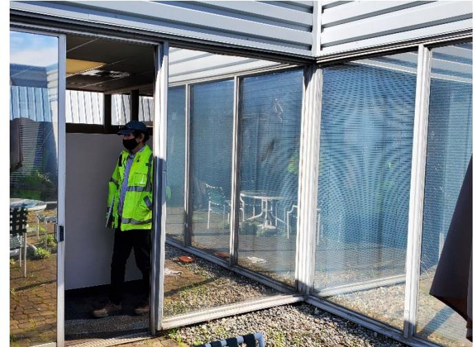
Figure 1 - Before construction, old leaky wood-trimmed windows and doors
