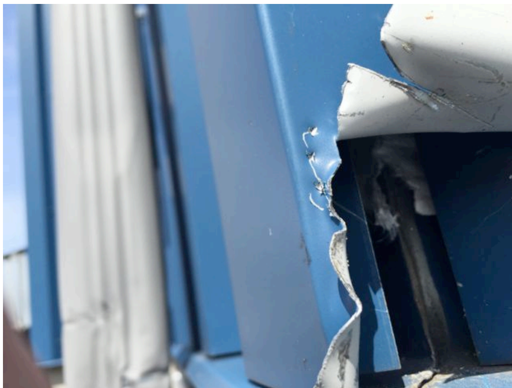
Photograph 11: Marine Building – Exterior Barrier under Metal Siding (Sample 1283-10A)
