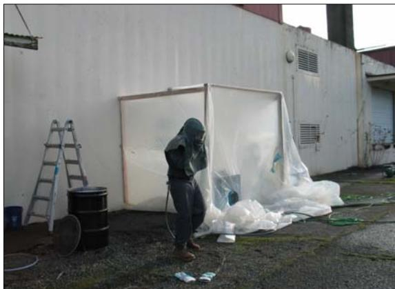
Exterior Blasting Containment System and Personal Protective Equipment
