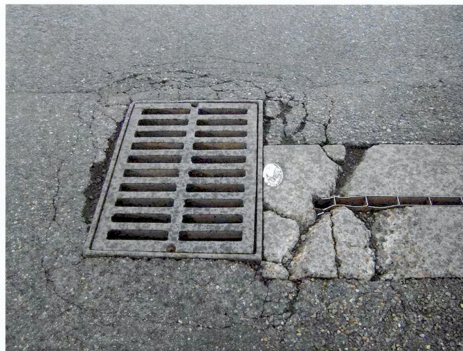
PHOTO - EXAMPLE EXISTING CONDITION
