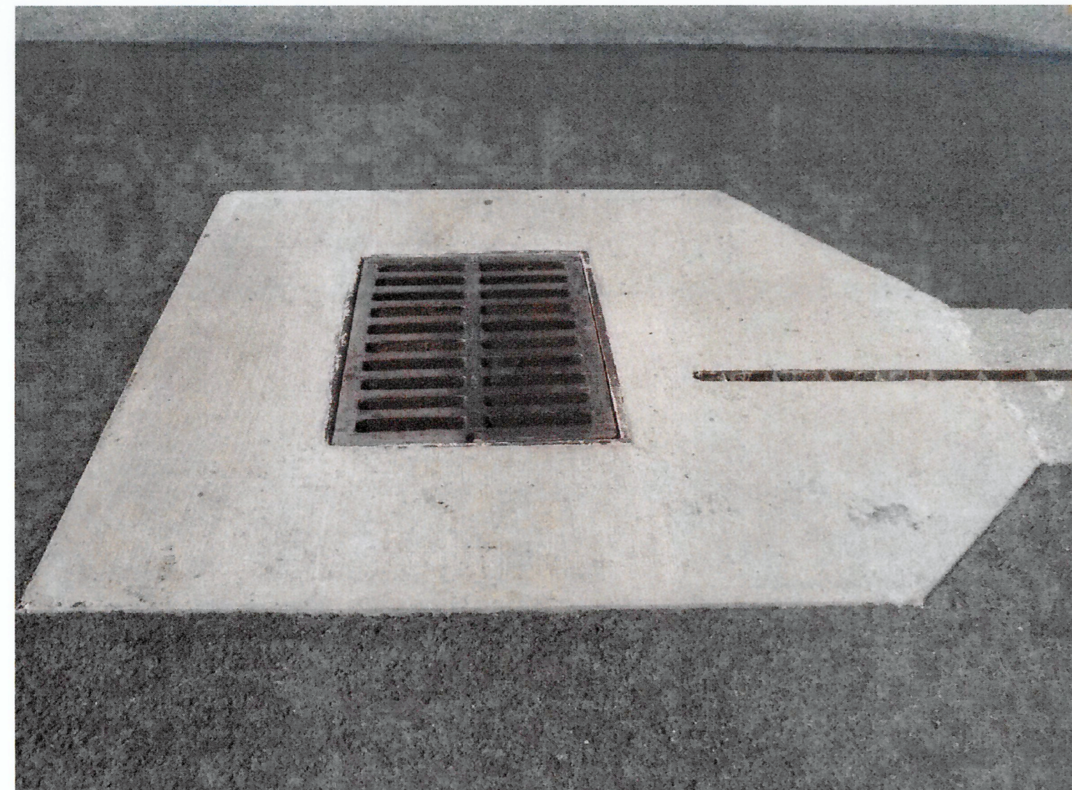
PHOTO - EXAMPLE FINISH CONDITION
