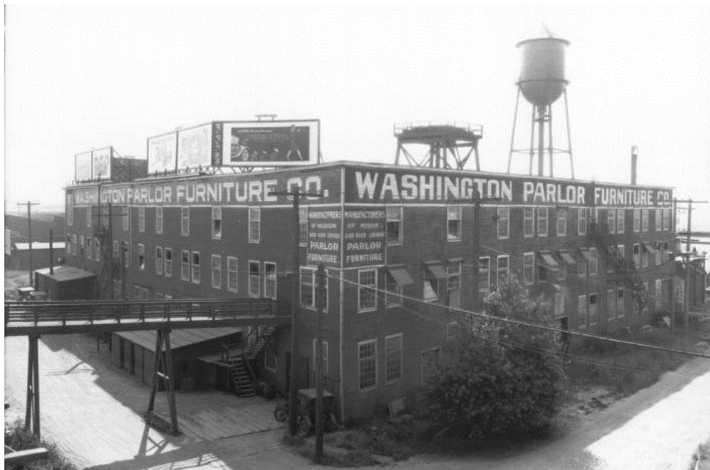
Photograph 6 (1930): View facing southeast toward the Washington Parlor Furniture Company building located immediately west of the Property.
