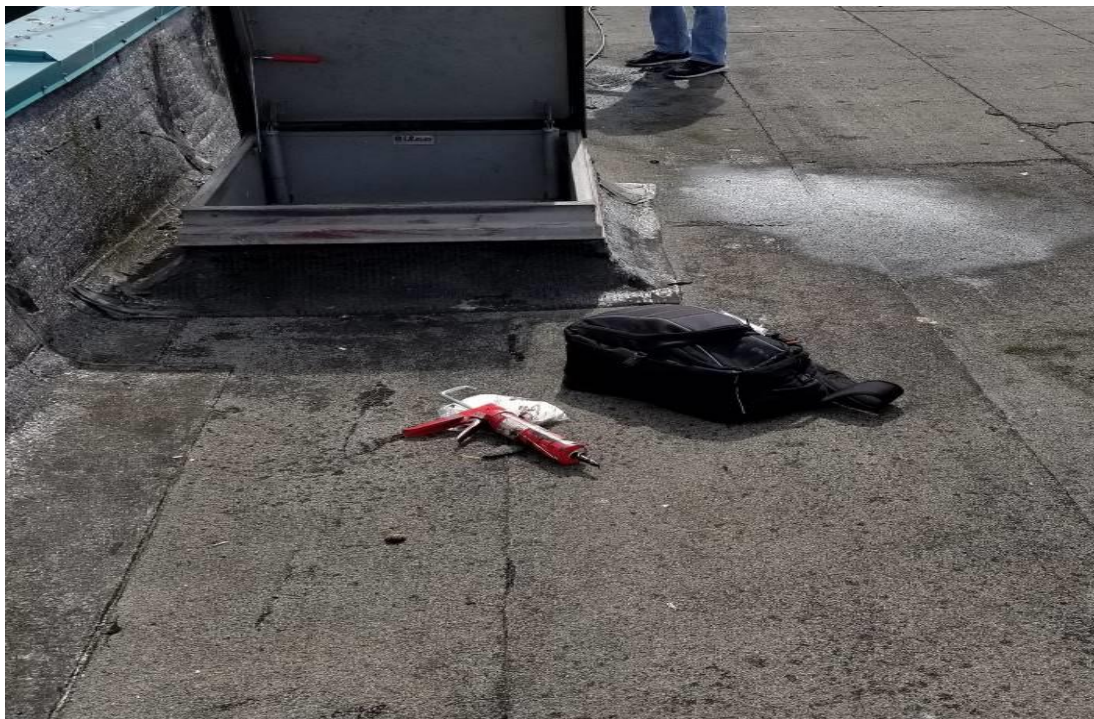
Photograph 7: Upper roof, sample 18 location, black mastic on base of ladder access unit.
