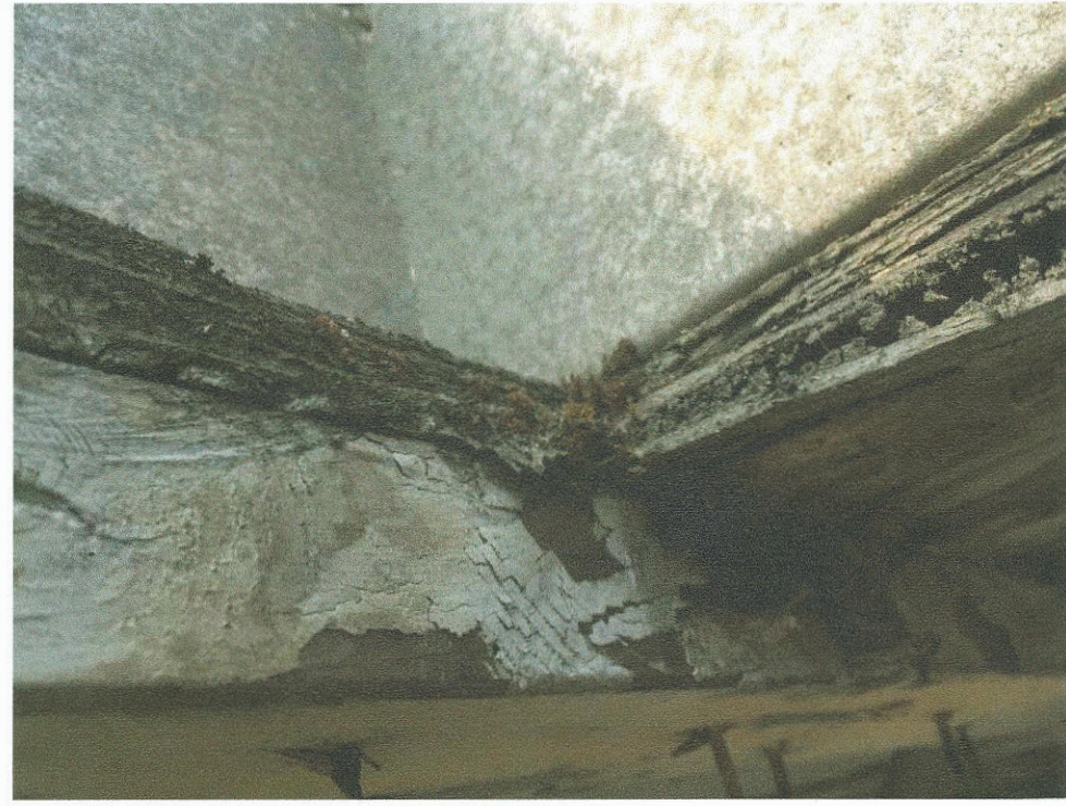
TYPICAL DAMAGE @ (E) SKYLIGHT
