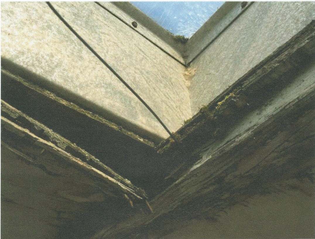
TYPICAL DAMAGE @ (E) SKYLIGHT
