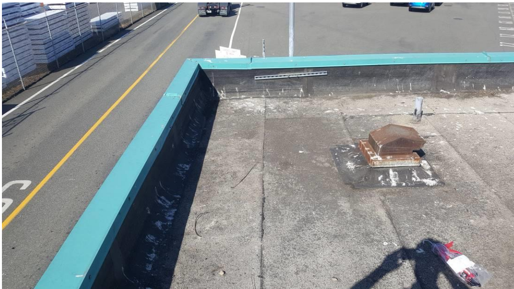
Photograph 3: Built-up roof system
