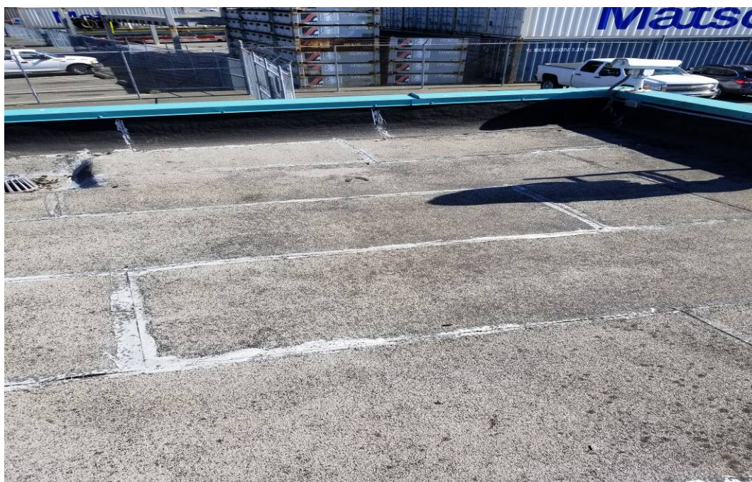
Photograph 2: Built-up roof system. All suspect materials were determined to be negative for asbestos.
