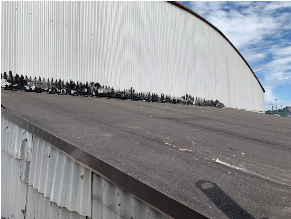
Photo 3: Roof of shed. The roofing is non asbestos containing.
