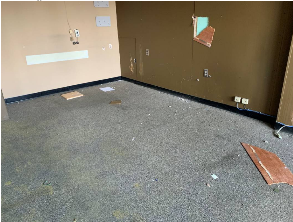
Photo 8: Typical finishes observed in the office area. The paneling mastic is ACM.
