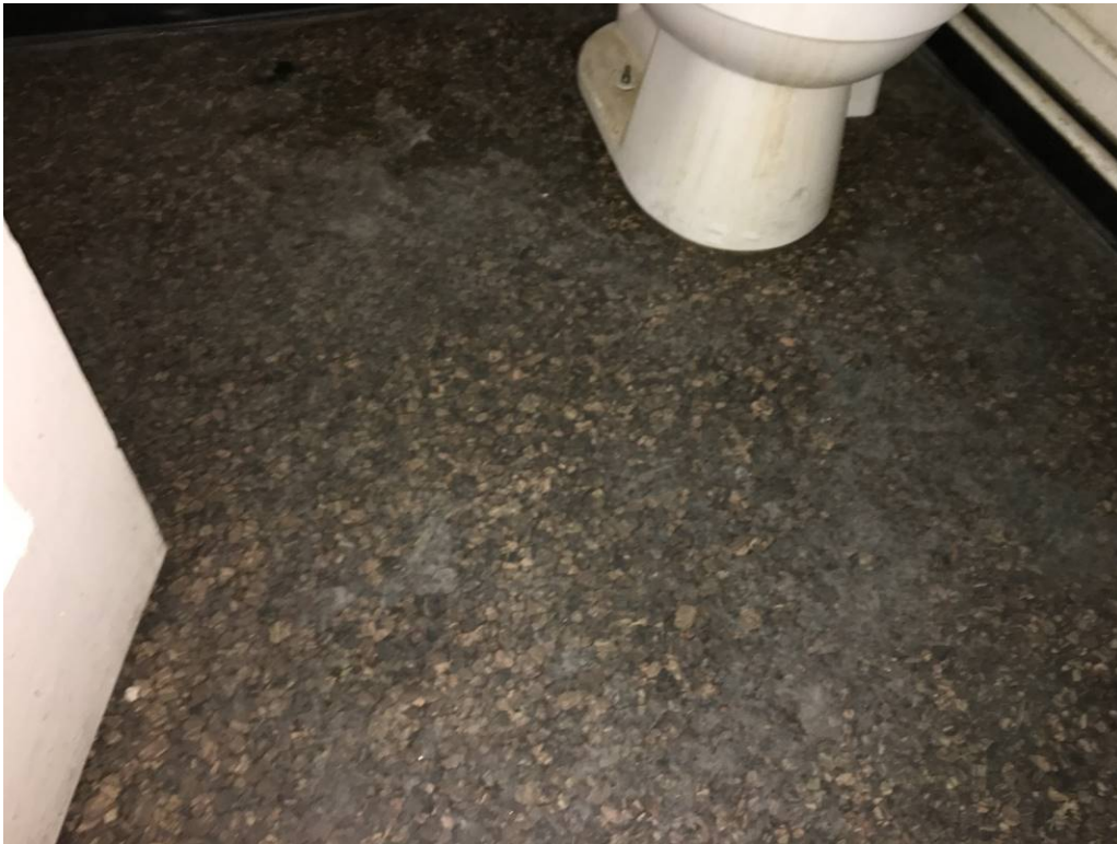
Photo 13: ACM flooring in the office restroom and storage area.
