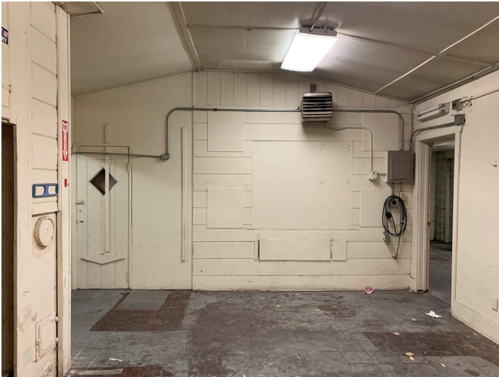
Photo 15: NE corner of the north section of the building the floor tile and mastic is ACM.
