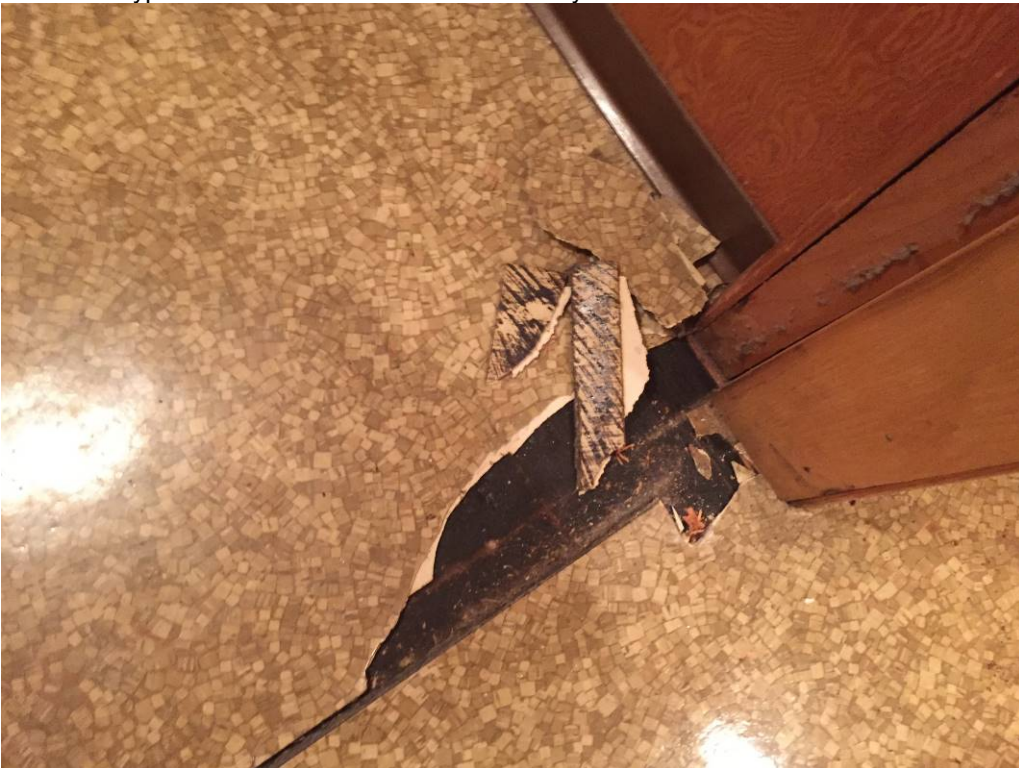
Photo 10: ACM AVF flooring and floor tile in the restrooms and closet. Rooms 16, 17, 19, 20, 24 and 25 only have ACM SVF.
