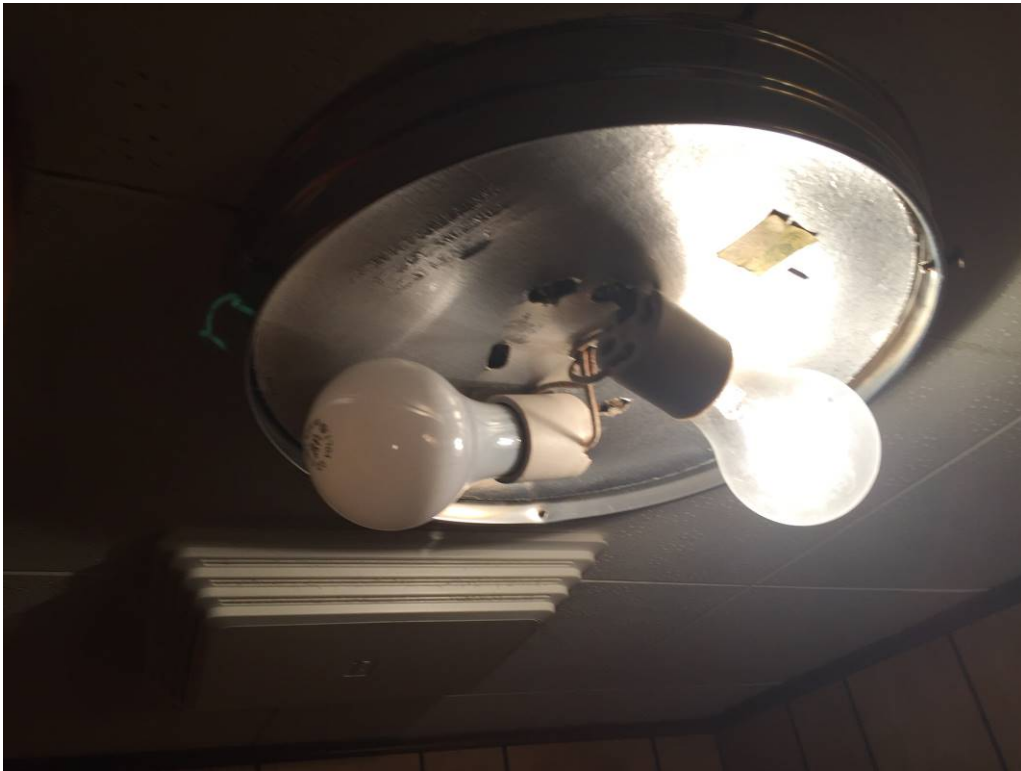
Photo 11: ACM light heat shields in restroom 5 and 6.
