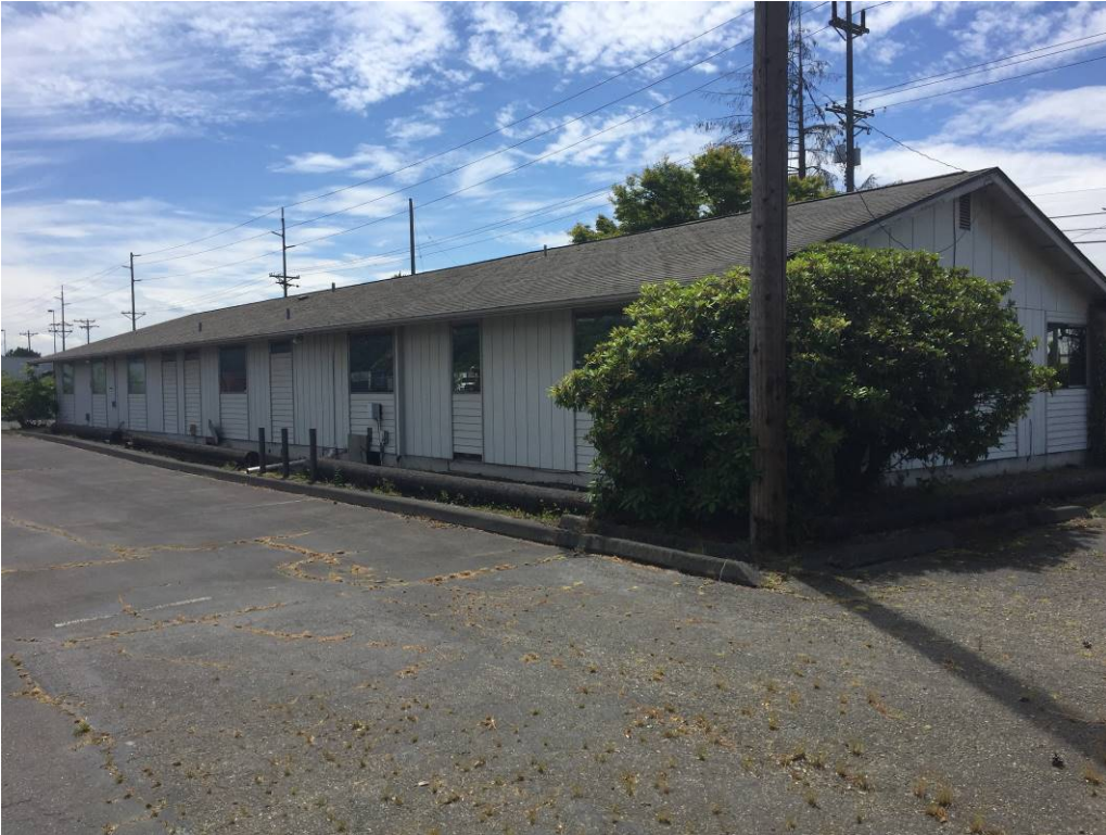
Photo 3: North side of the building facing southeast. The skirting around the perimeter is CAB.
