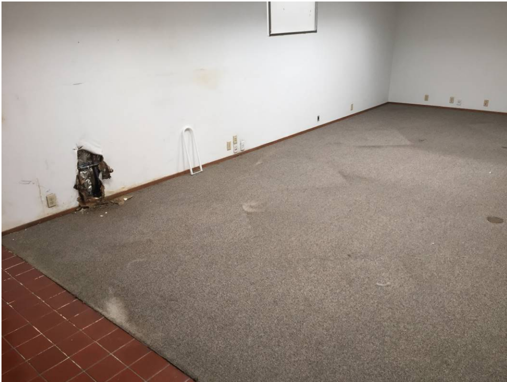
Photo 13: Typical finishes observed in the office spaces. The orange peel textured GWB system was determined to contain <1% asbestos. This material is located throughout the building.
