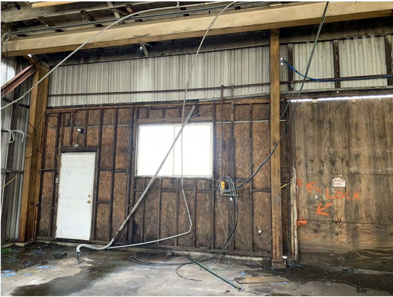
4 PHOTO - INTERIOR ELEVATION N1 NTS
