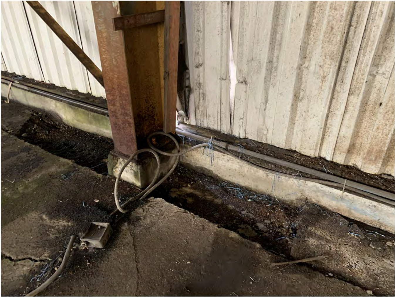
3 PHOTO - INTERIOR VIEW NTS
