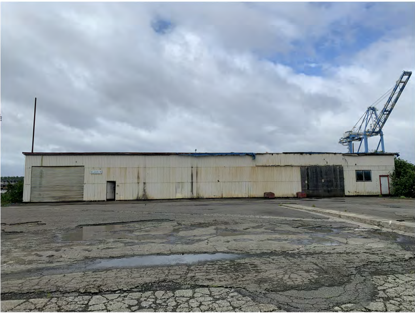
1 PHOTO - EXTERIOR ELEVATION N NTS
