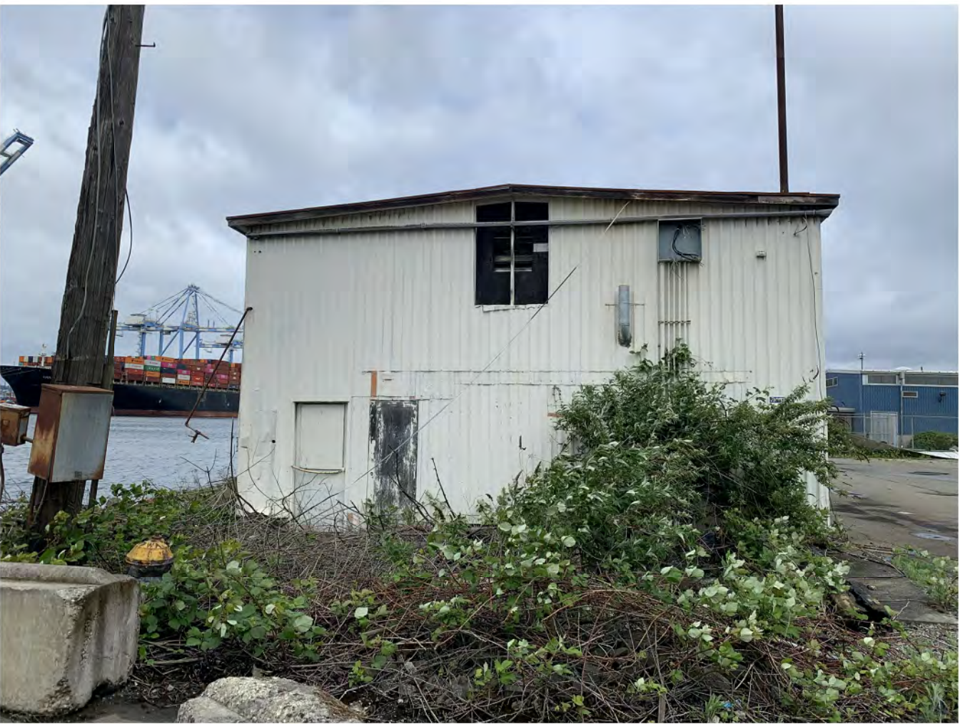
2 PHOTO - EXTERIOR ELEVATION E NTS
